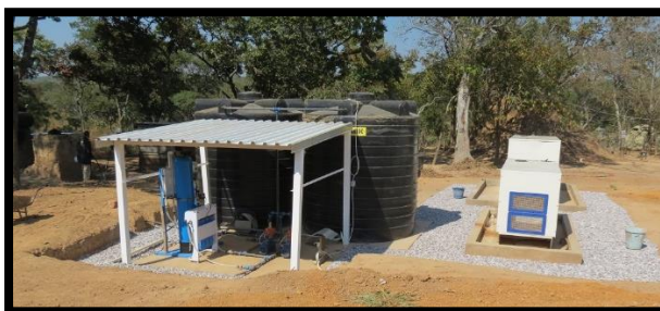
New water storage/filtration and gensets
