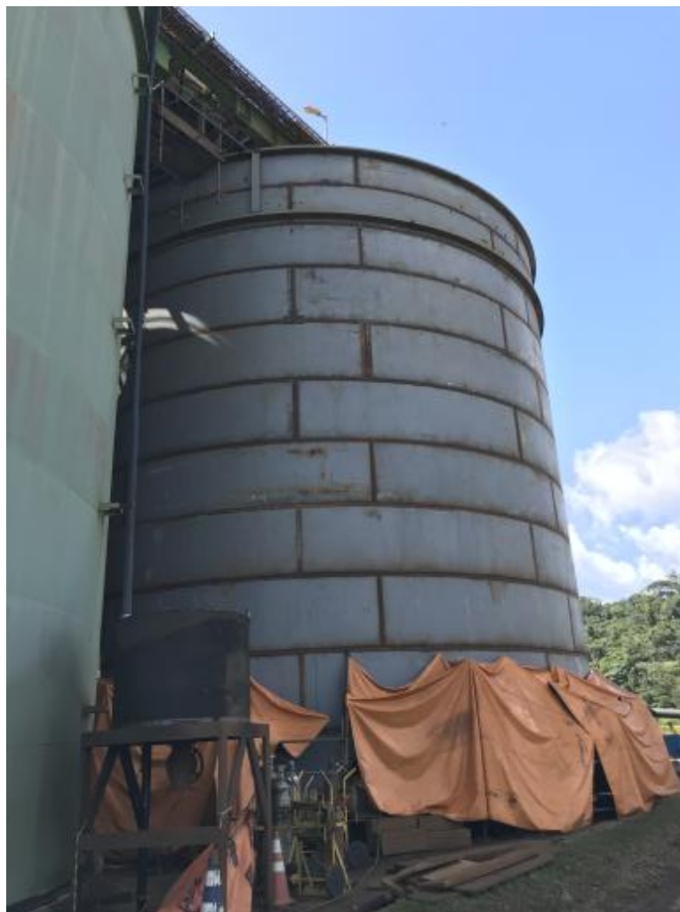
Figure 6. CIL Tank - erection completed
