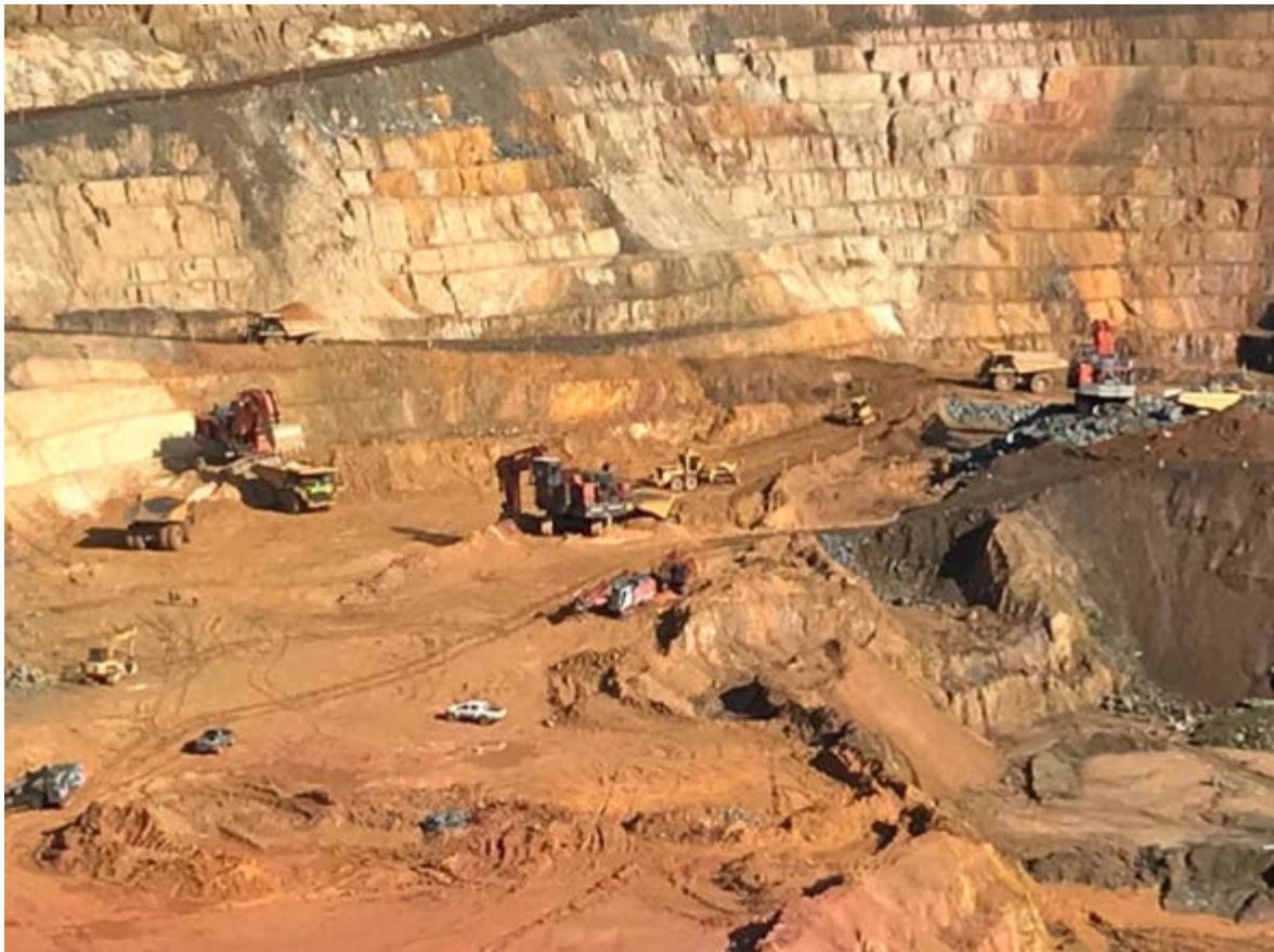
Figure 10. Three U&M Excavators operating at TAP AB
