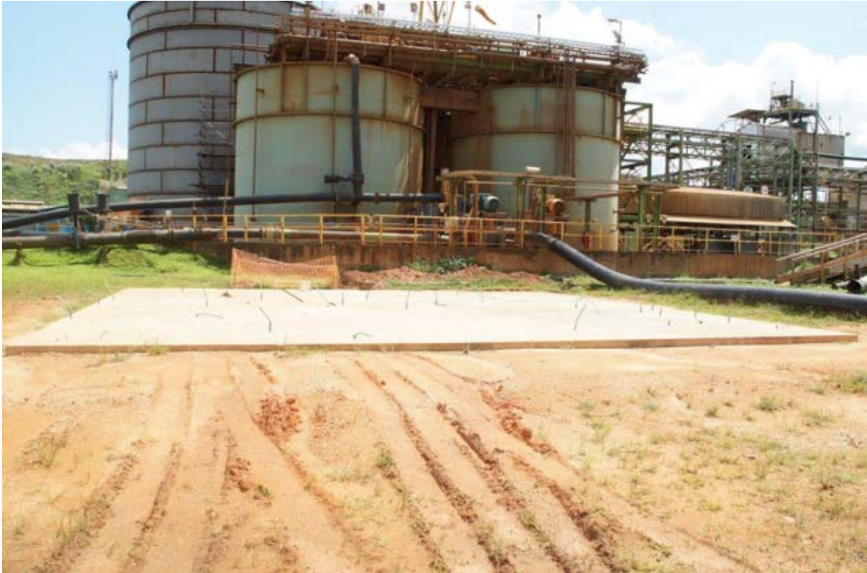
Figure 8. Oxygen Plant – Concrete Pad Completed
