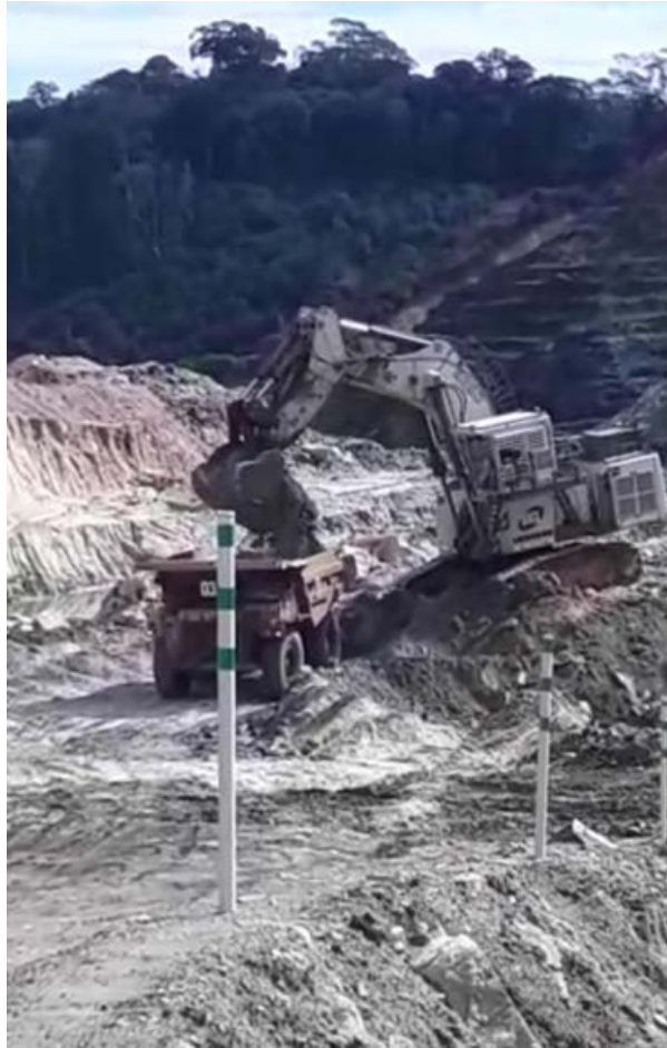
Figure 9. Excavator operating at Urucum
