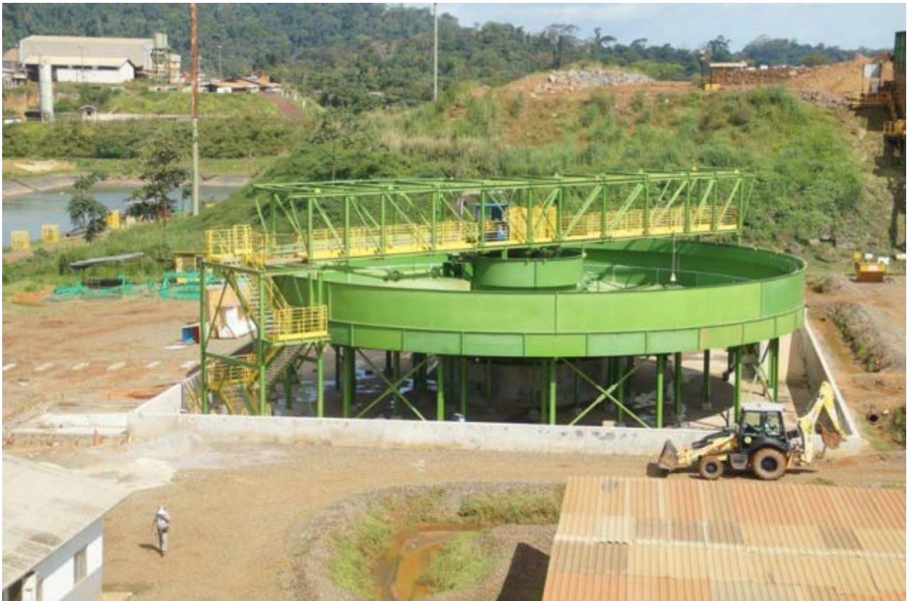
Figure 4. Pre-Leach Thickener – external construction completed
