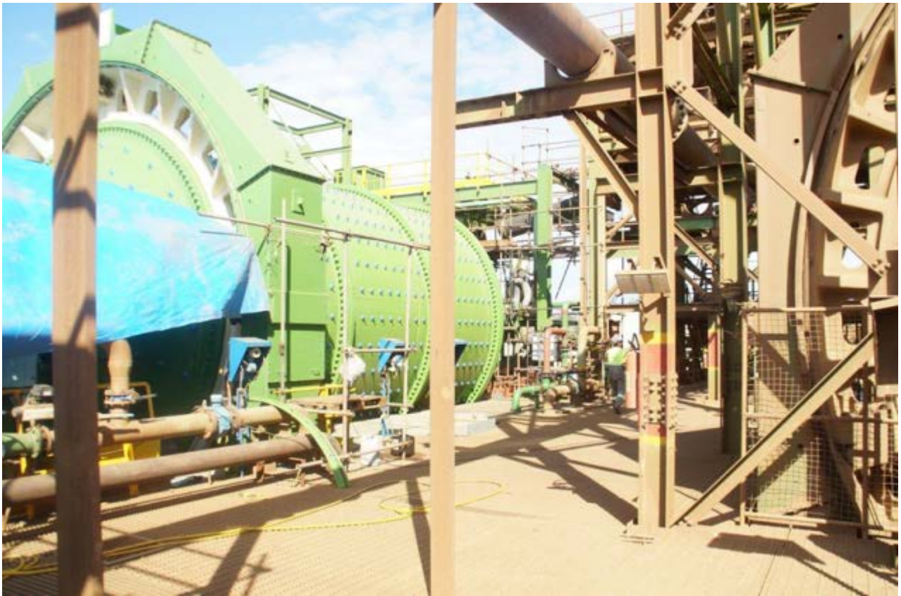
Figure 2. Ball Mill – Installation of rubber lining system completed
