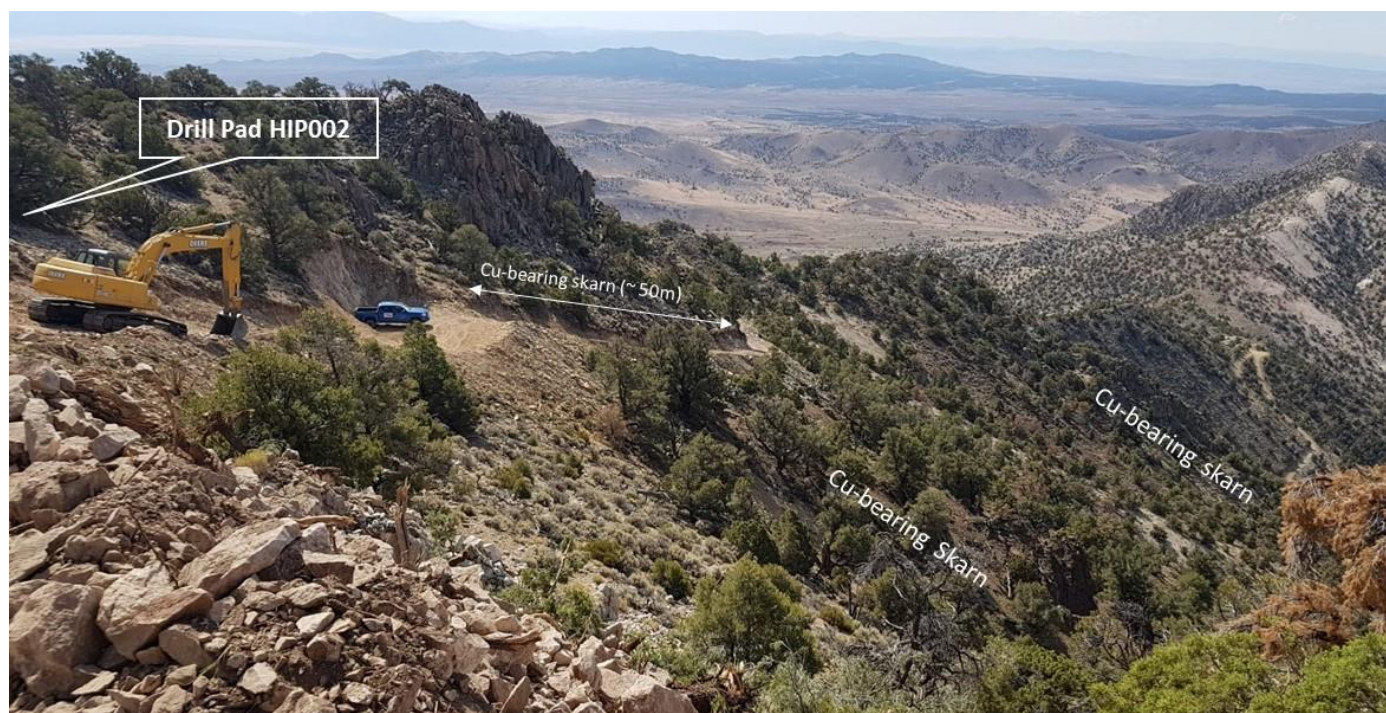
Figure 1: Roadworks and drill pads nearing completion. At least seven drill holes for up to 3000m are planned from drill pads HIP002-HIP004 along the Upper Accrington road as part of an overall 7000m program.
