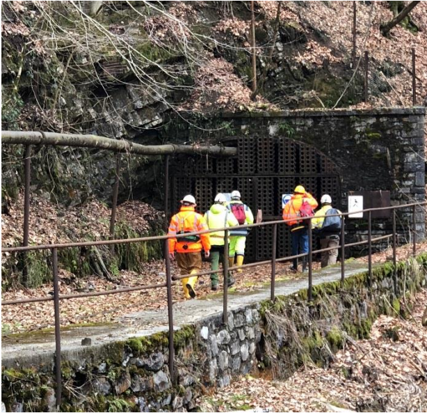
Figure 3: Entry to the Riso-Parina tunnel
