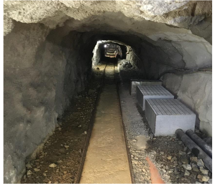
Figure 4: Interior view of Riso-Parina tunnel
