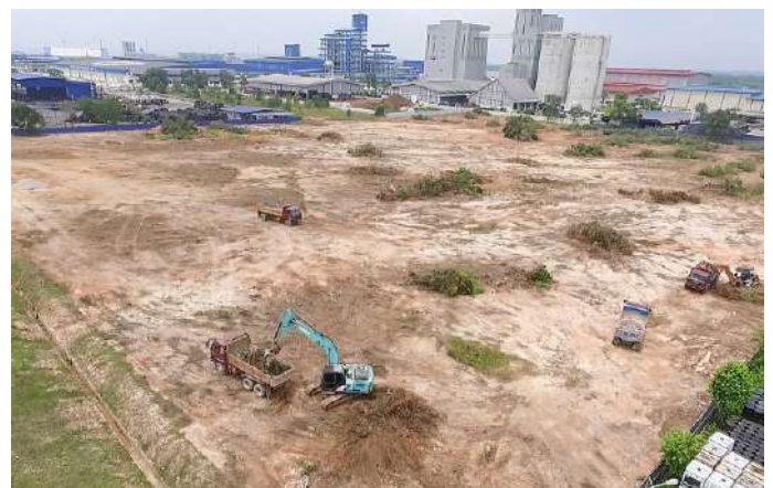
Figure 4. Completion of site clearance work at the Johor HPA site
