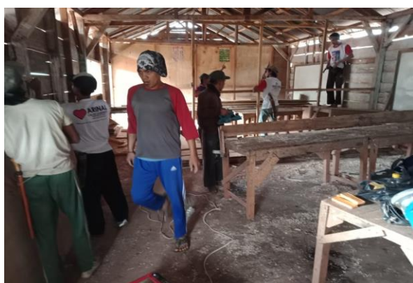
Figure 5: Building maintenance of elementary school in a local village
