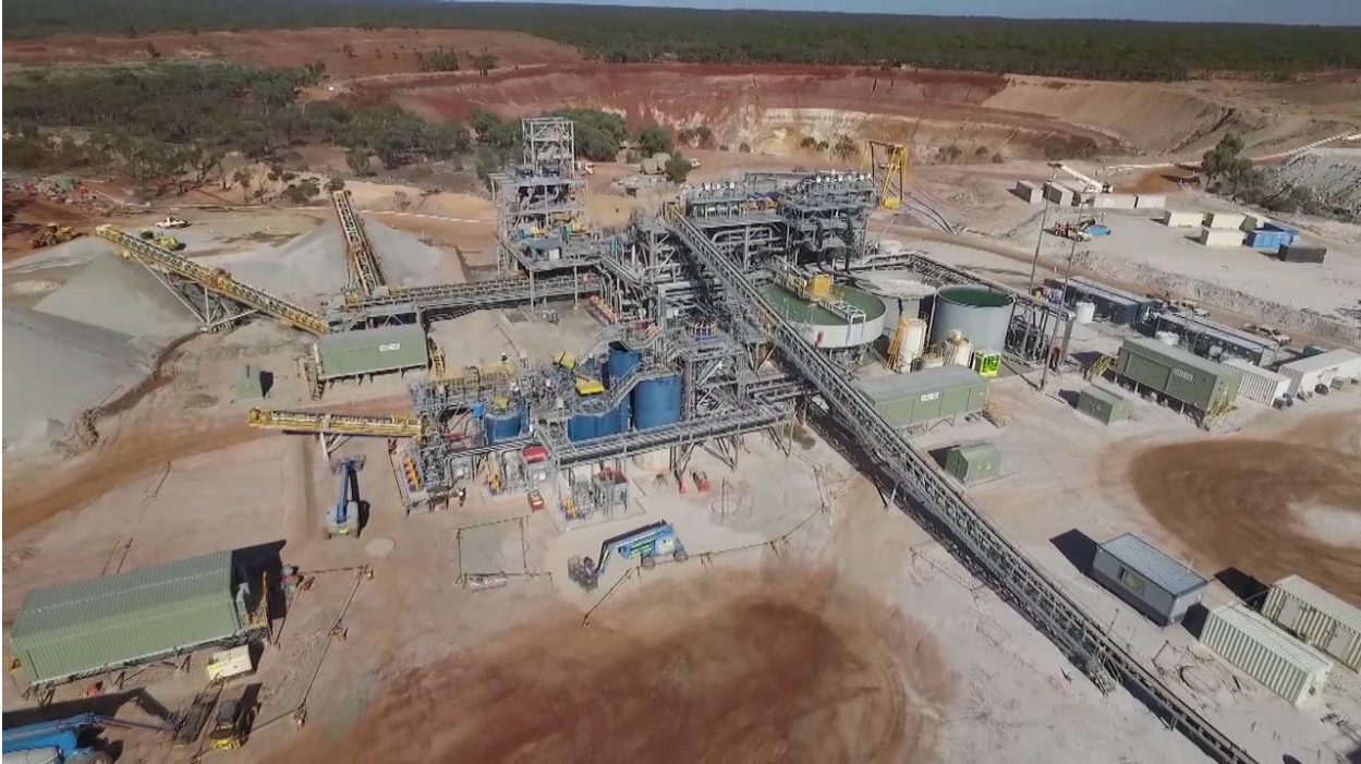
Image 1 - Aerial View of the Mt Marion Lithium Operation Processing and Tailings Storage Facilities
