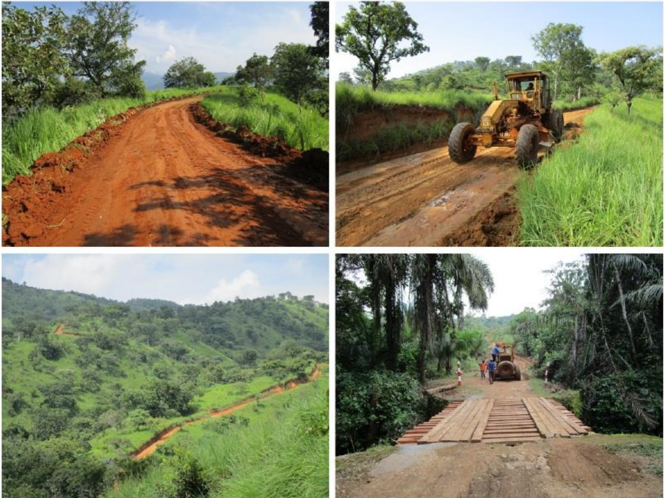
Figure 3: Road and bridge upgrades for drilling rig access on the Mayouom Project
