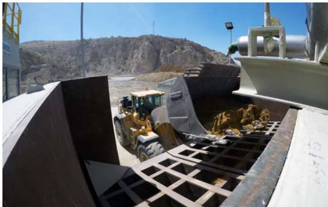
First oxide ore test into crushing circuit
