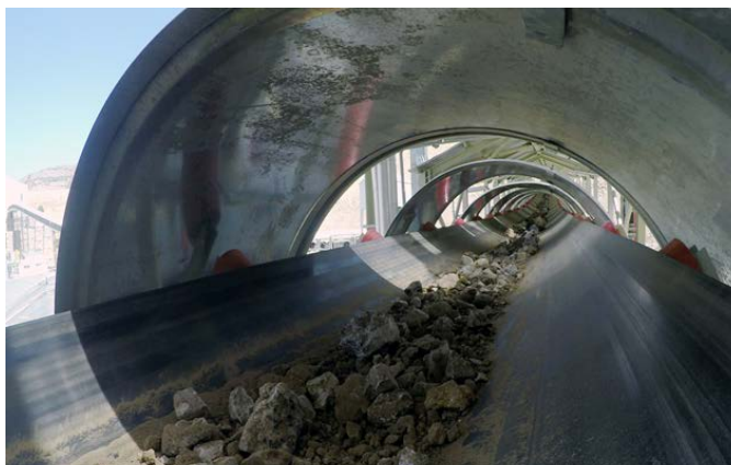
First oxide ore test on conveyor
