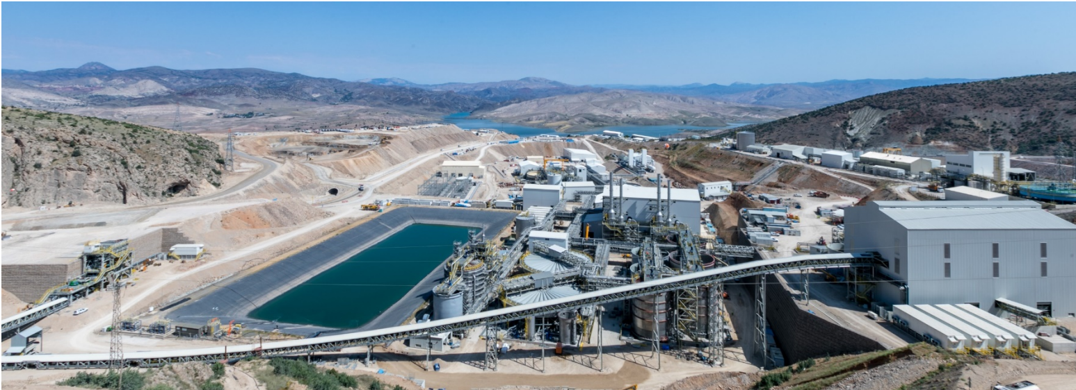
Overview of the Project Site
