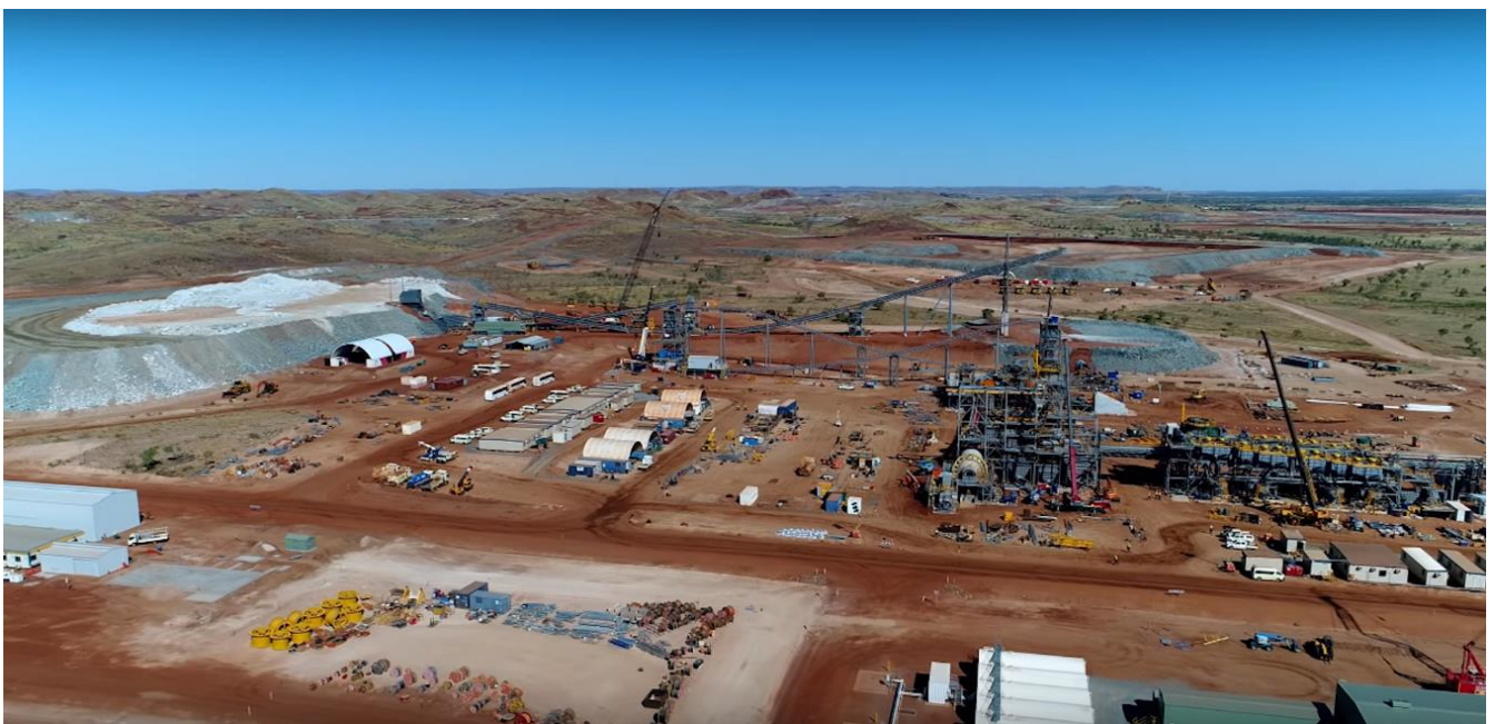
Figure 2: Aerial photograph of Stage 1, 2Mtpa project construction
