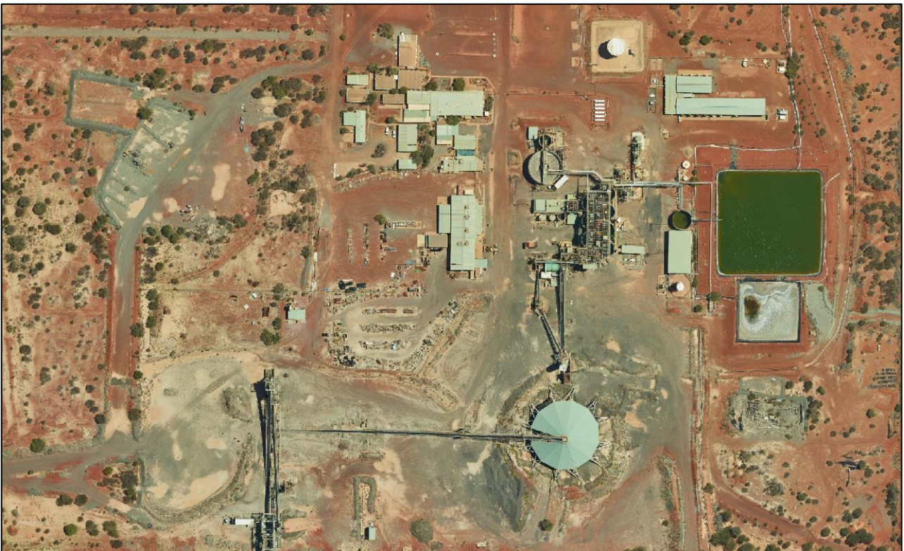
Figure 7: Bronzewing Process Plant
