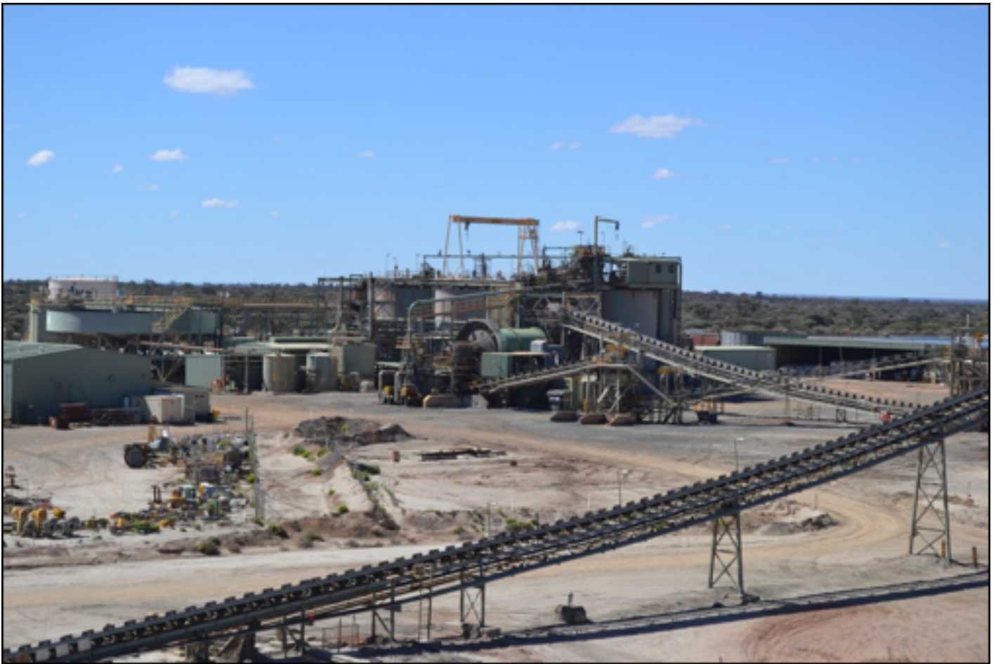
Figure 1-11 Bronzewing Processing Plant
