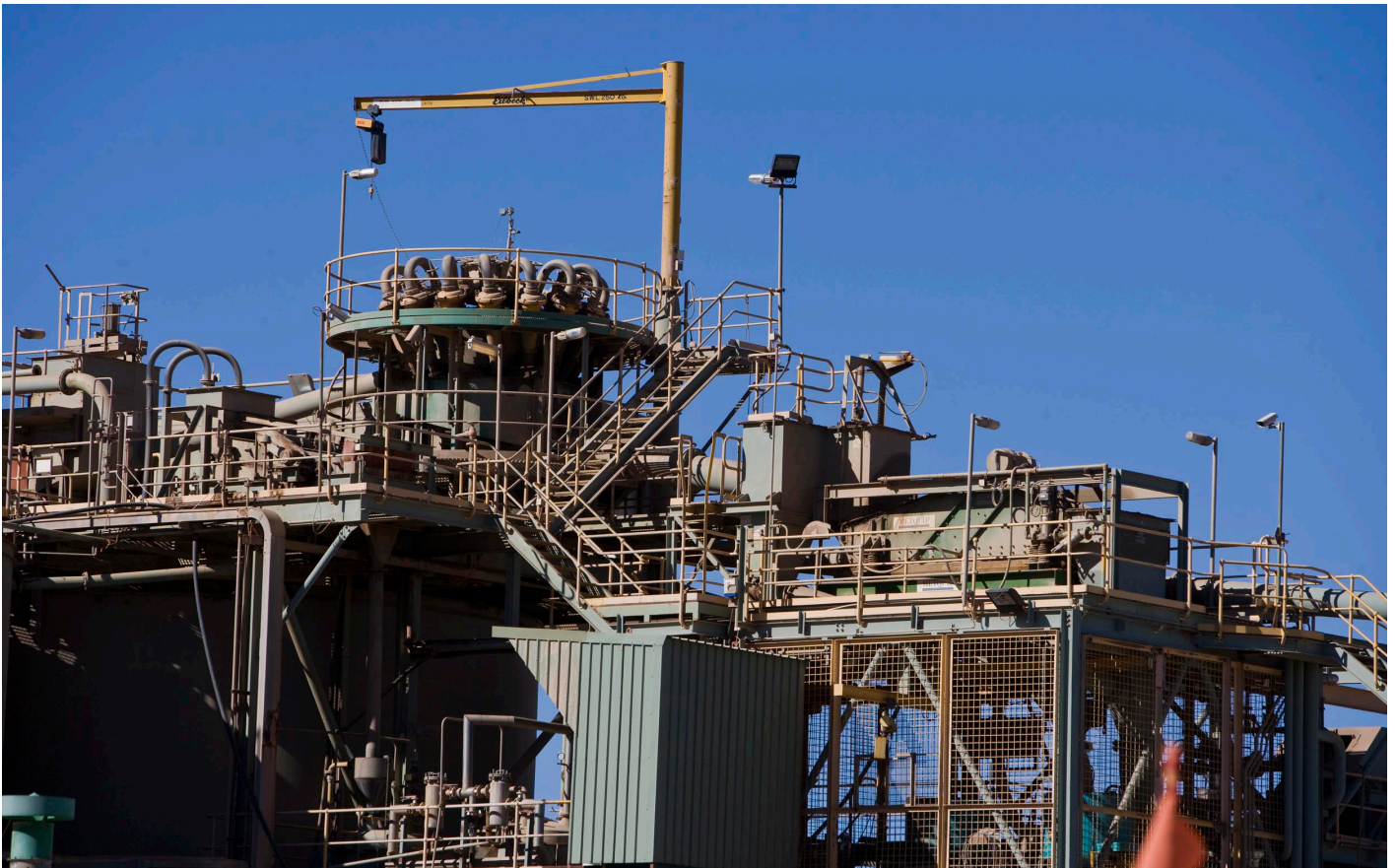
Figure 1-1 Bronzewing Processing Plant
