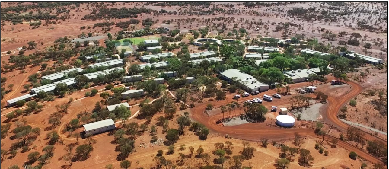
Figure 8: Bronzewing Accommodation Village
