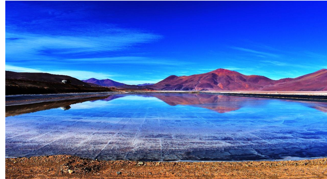
Rincon Project – Stage 2 Evaporation Ponds
