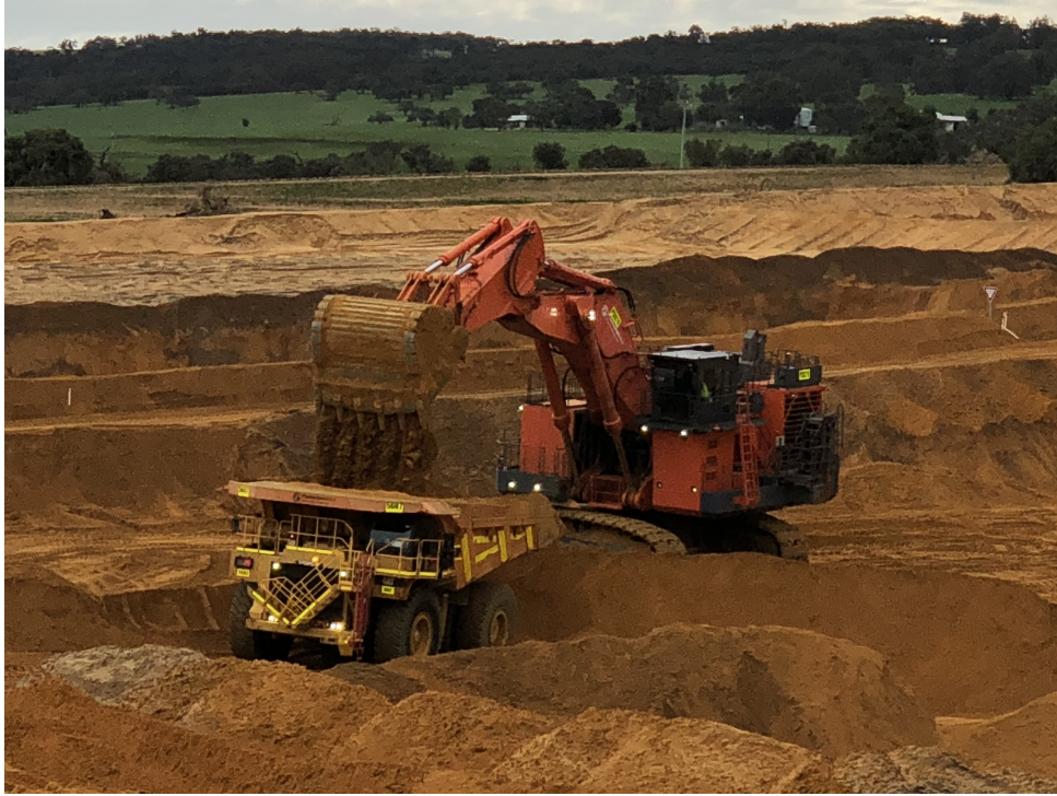
Photo 3: Hitachi 3600 Excavator and CAT 785 truck
