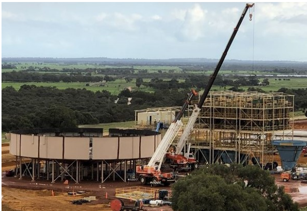
Photo 1: WCP construction looking northwest
