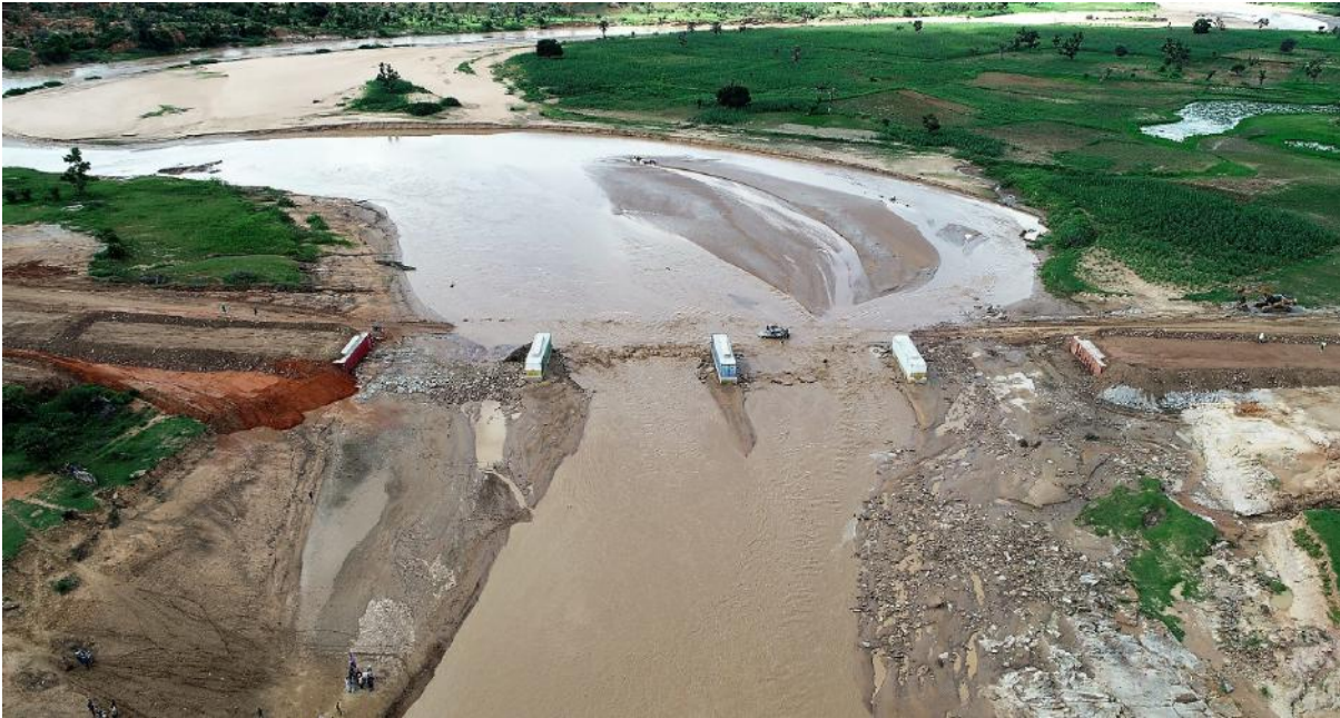
Image 4: Completion of Bailey bridge
