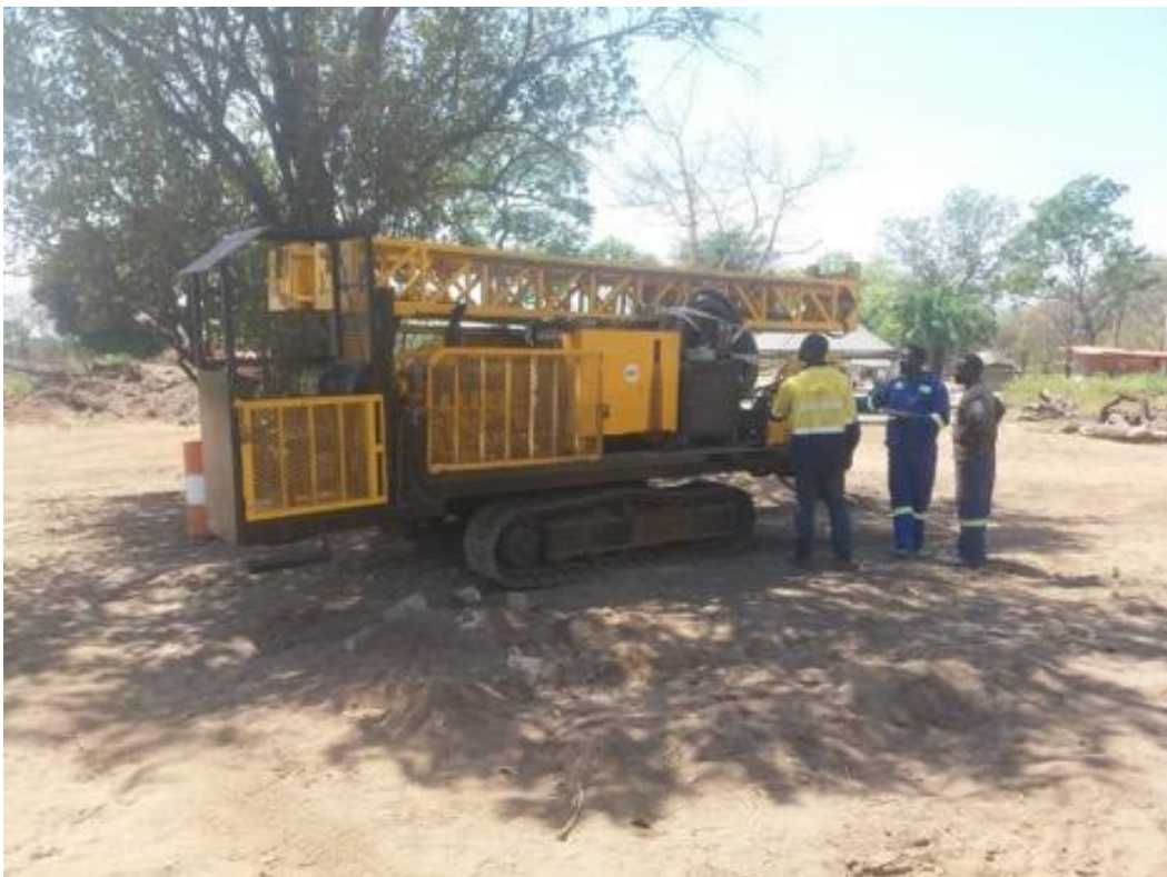
Figure 8: Diamond Drill Rig at the Kanuka Lithium Production Project in the DRC
