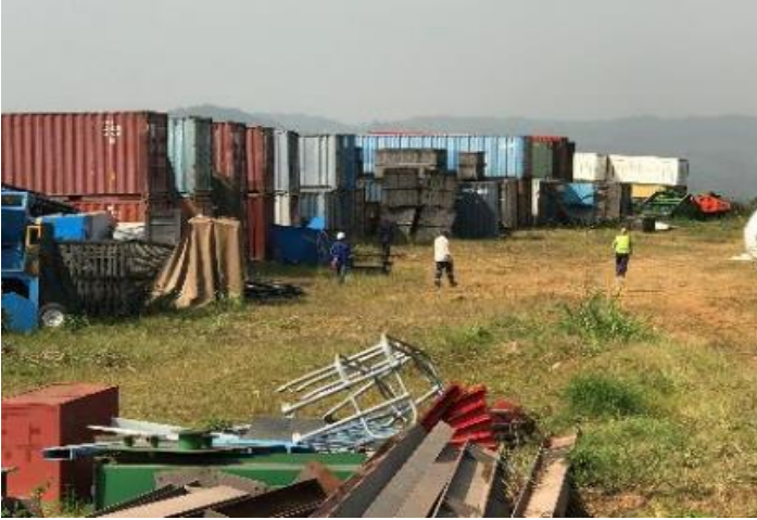
115 containers at site
