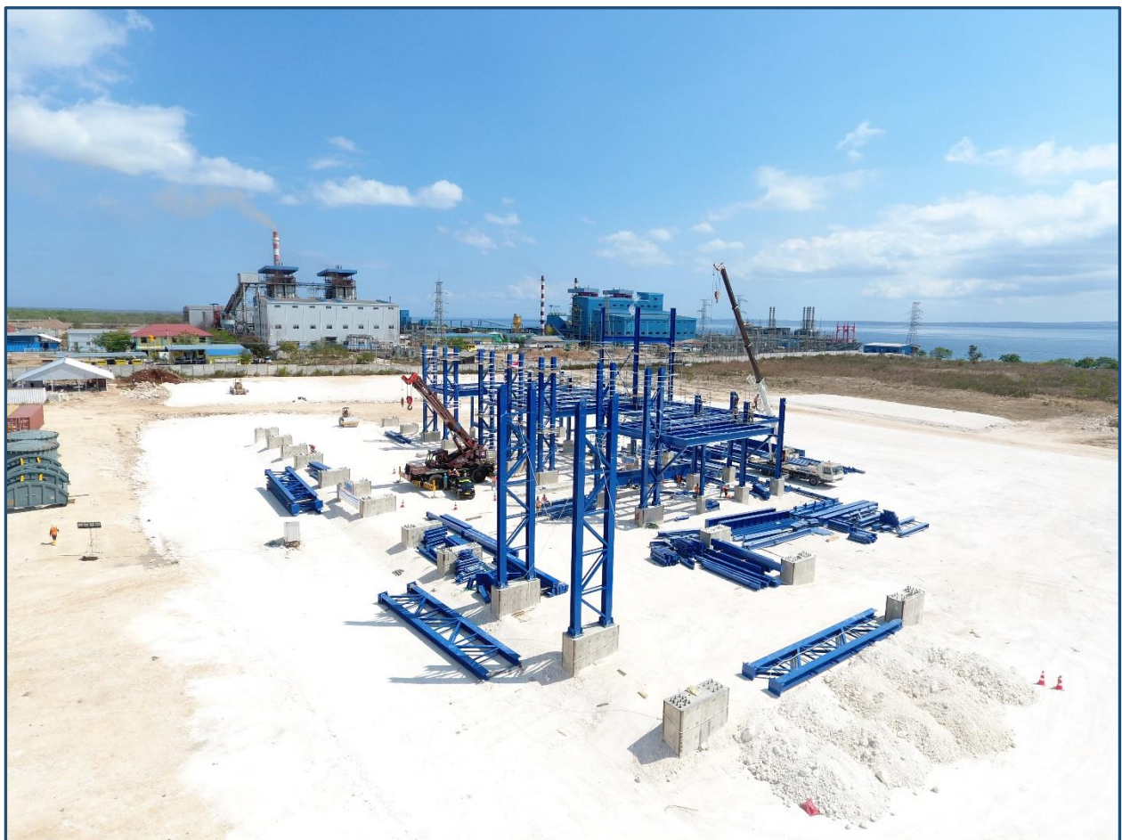
Figure 1: Construction progress at Gulf's Kupang Smelting Facility.
