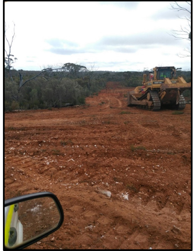
Photo 3: clearing the surface over the open pit
