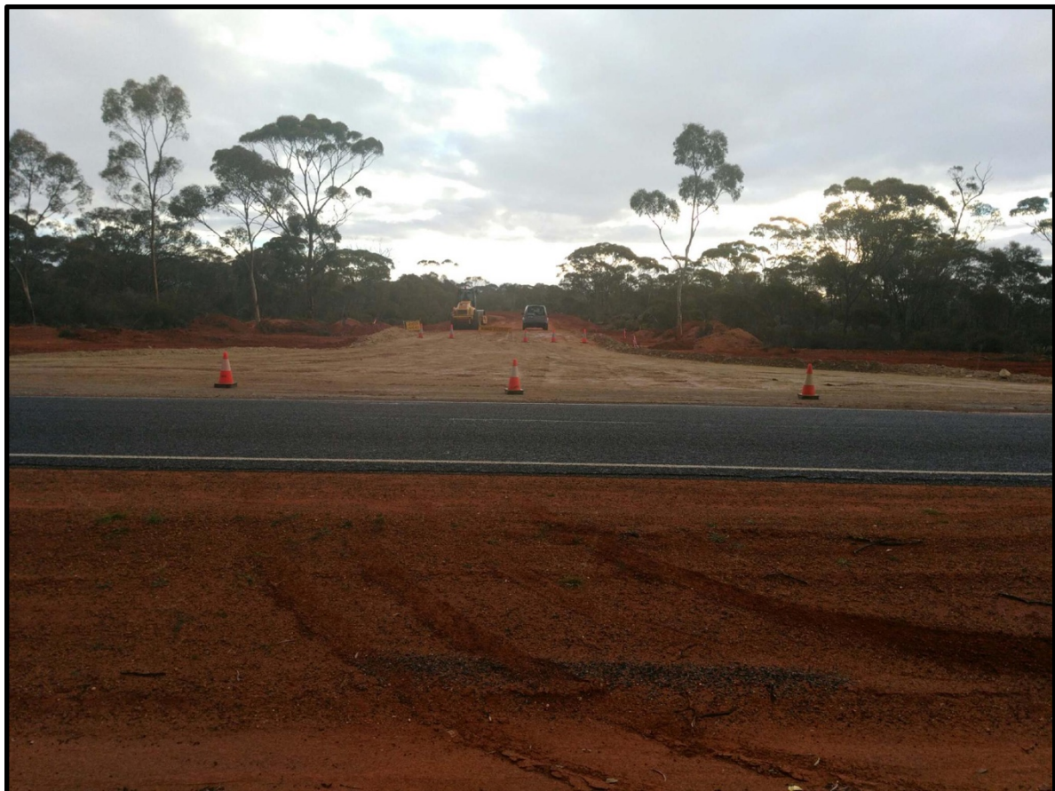
Photo 1: Construction of the Site access road
