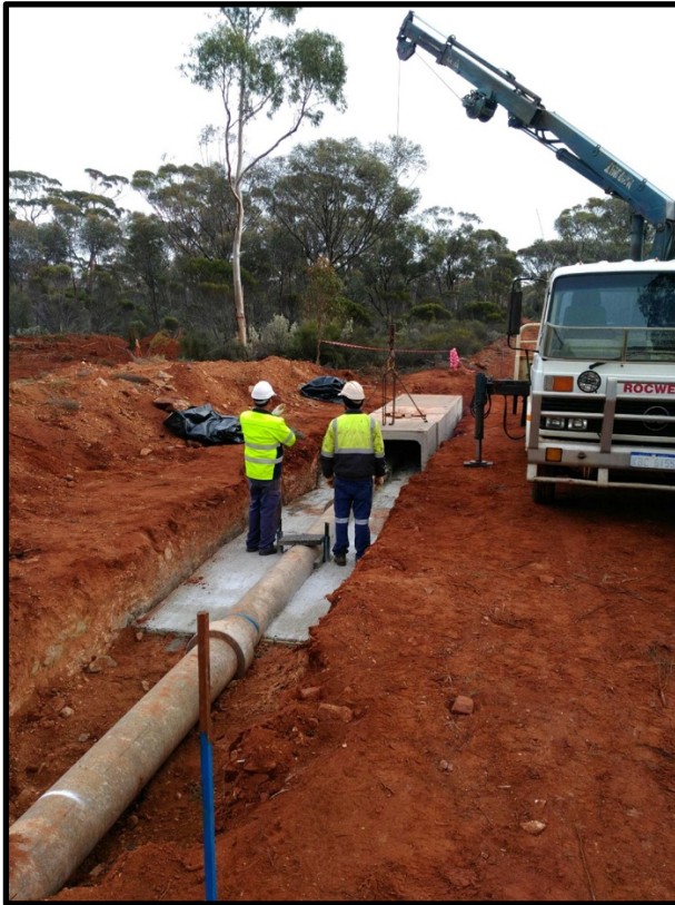
Photo 2: Access road culvert
