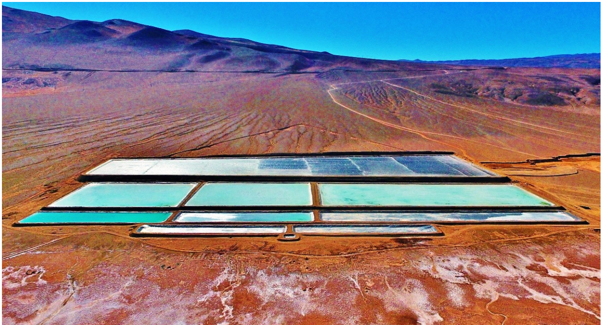
Figure 1. Rincon Lithium Project – Current Stage 2 Evaporation Ponds, additional 9 hectare pond (at top)
