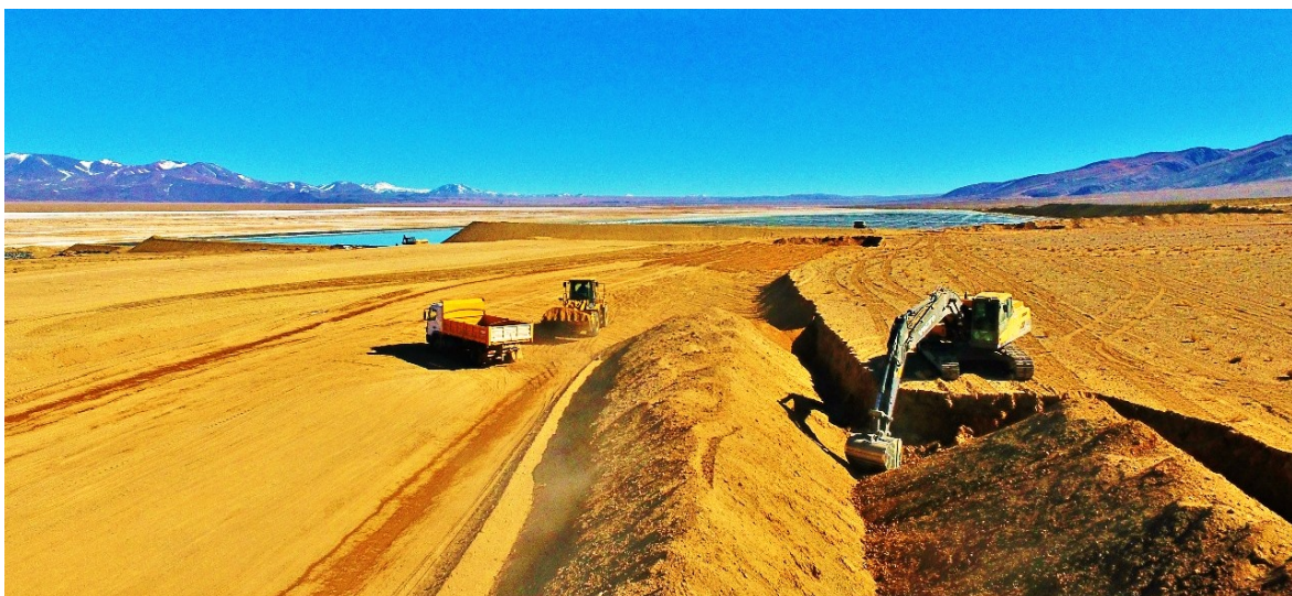
Figure 3. Rincon Lithium Project – Ongoing Stage 2 Evaporation Pond Construction Works Progressing
