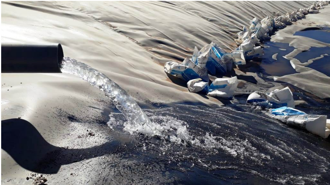
Figure 2. Rincon Lithium Project – Lithium Brine Pumping into Additional Stage 2 Evaporation Pond
