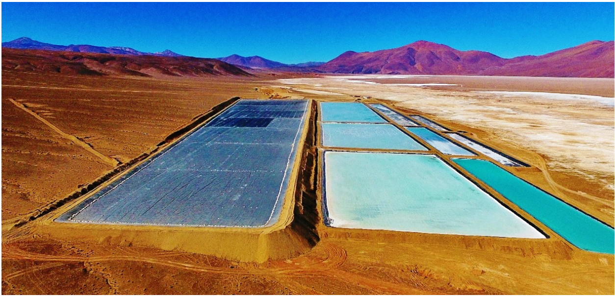
Figure 4. Rincon Lithium Project – Current Stage 2 Evaporation Ponds → Additional 9 Hectare Pond (on left)
