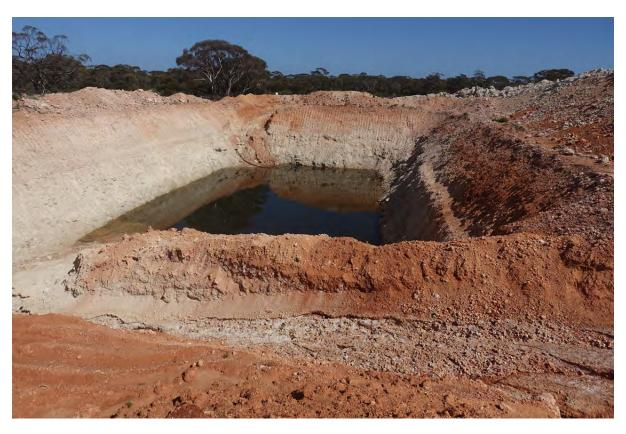
Figure 2: Walls within the Cammi's Creek Pit remain stable following formation of Pit Lake (looking west)
