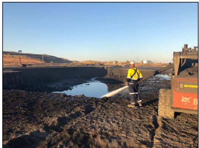
Figures 4 & 5: Hydraulic miners cutting in the initial channel near the inlet to the Slurry Winning Pontoon
