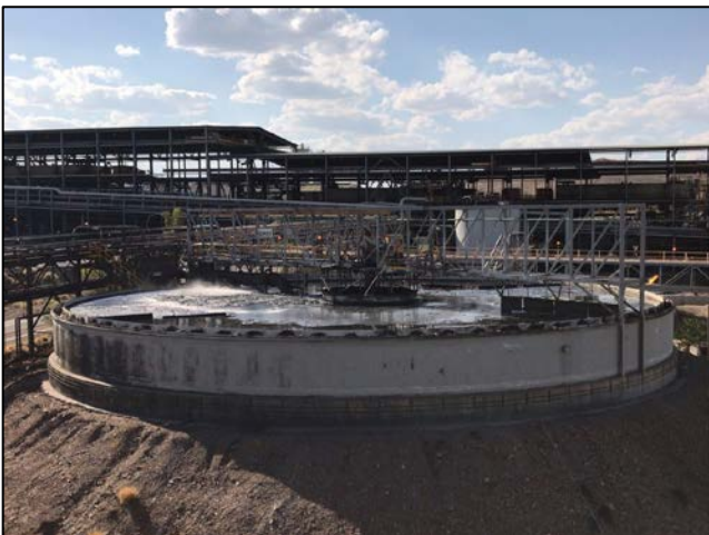
Figures 10 & 11: Zinc Product Thickener filling with final concentrate at the Lawn Hill mine site in preparation for transit up the pipeline to Karumba (left) & deposition of final tailings into the historical open pit (right)
