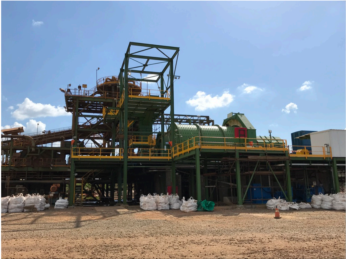
Figure 2. View to operating ball mill
