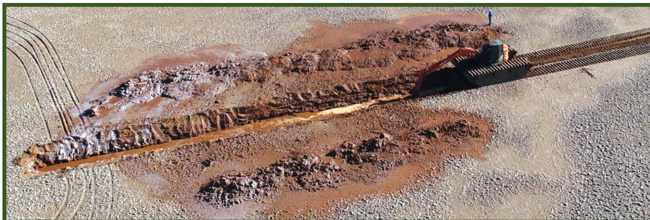
Figure 8: Trench SENE in construction
