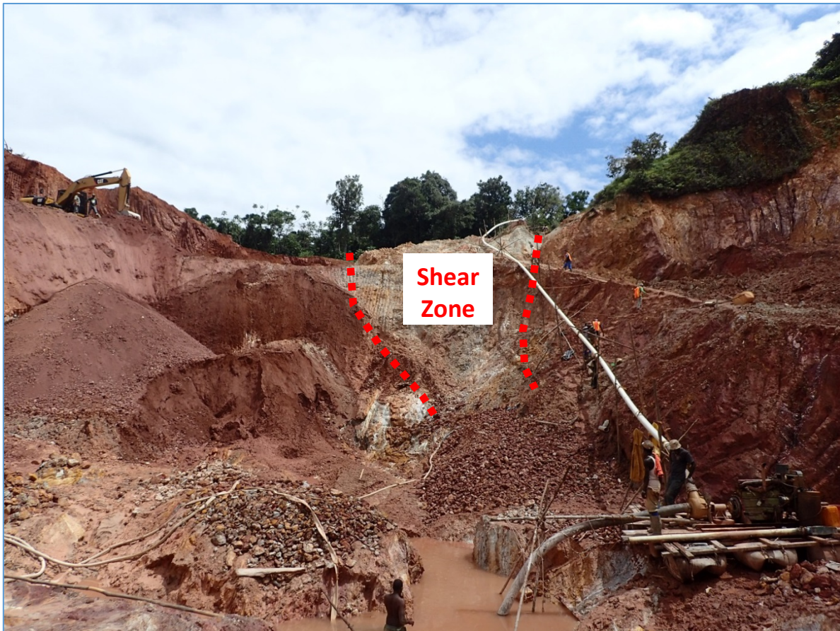
Figure 3: Artisanal mining operations in the Tallman pit, Ohio Project, looking south
