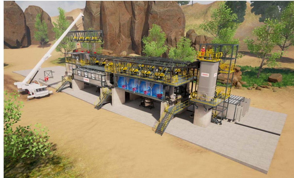
Image source: Outotec. cPlant Flotation showing modular construction .
