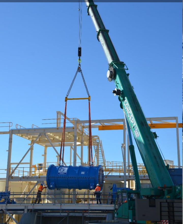
M10000 3MW 'Cameron Brown' unit being craned into position
