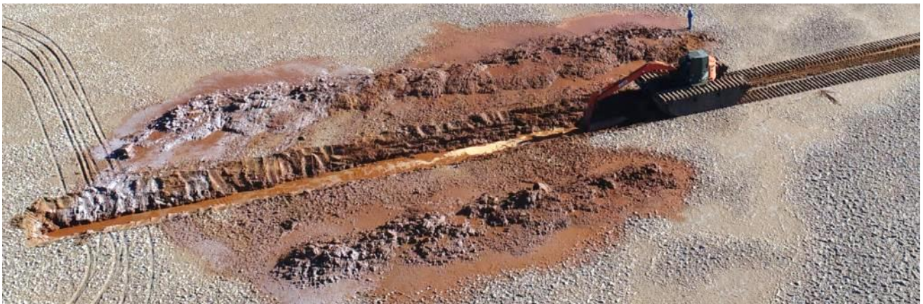
Figure 22: Trench SST02 in construction [12]
