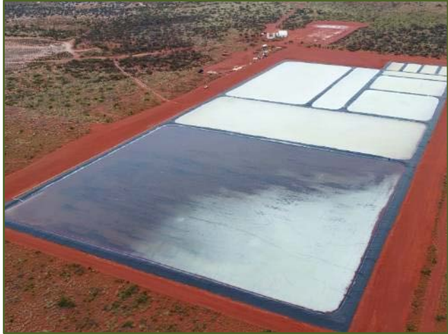
Brine Solar Evaporation Located in high evaporation region
