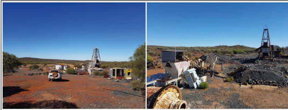
Figure 4-14: Photographs of Reid's Ridge historic mine, including headframe, crushing circuit and processing tanks
