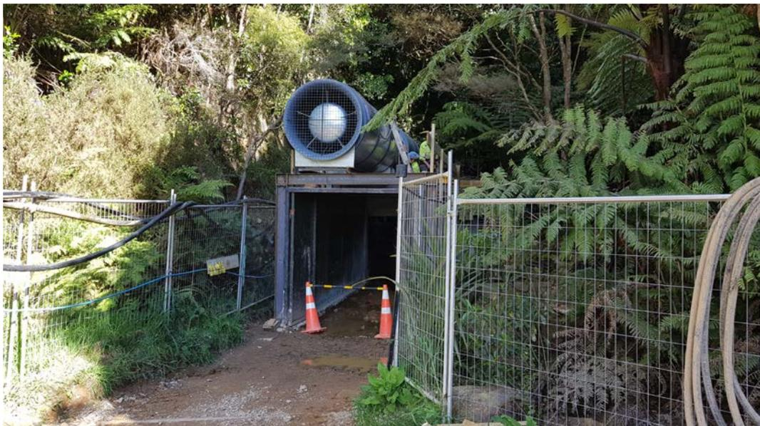
*Figure 2 - Main Fan in position above the airlock*
