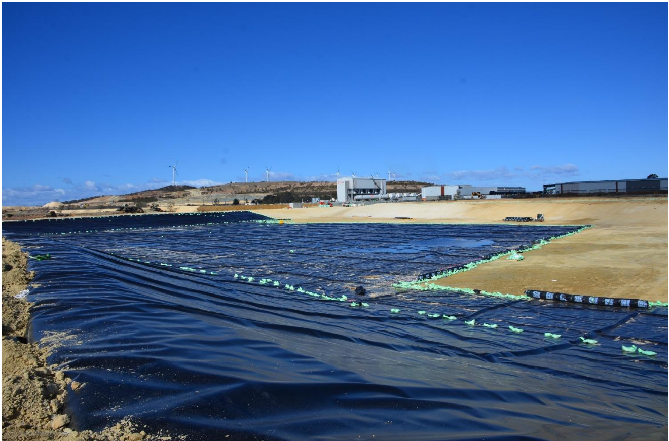
Figure 9: Lining of evaporation dam – cell 3 (1 August 2018)
