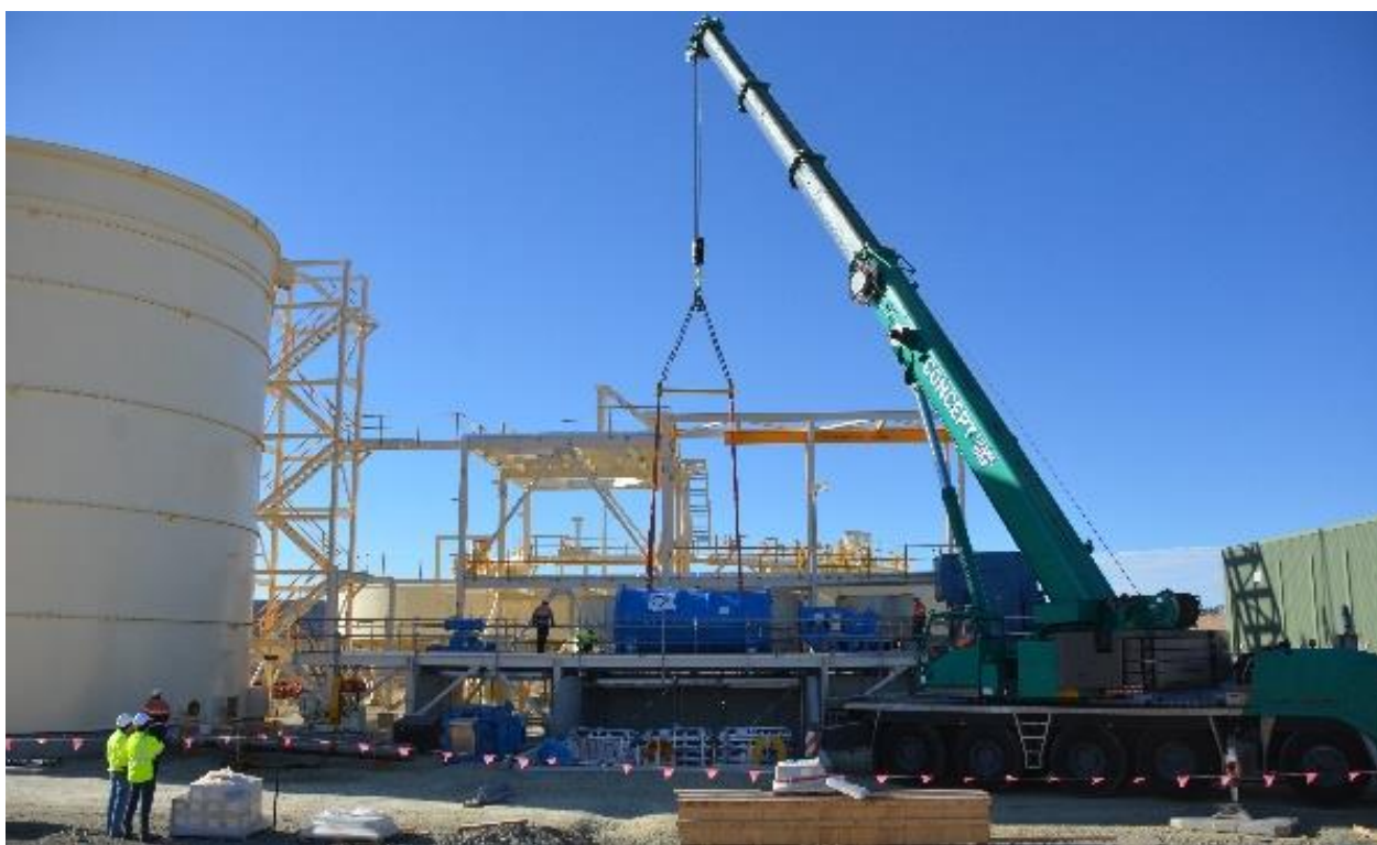
Figure 6: IsaMill installation (15 August 2018)
