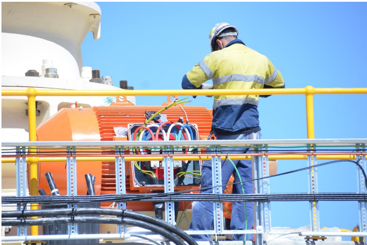
Figure 5: Secondary (cone) crusher electrical connections (13 September 2018)
