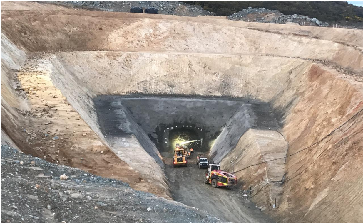
Figure 1: The first portal development firing to access the high grade underground resource (23 September 2018).
