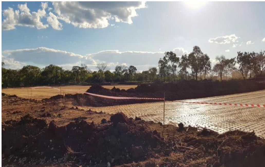
Plant site works
