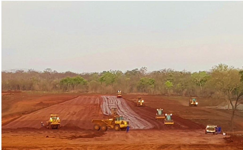
TSF civils work adding 2500 bcm/day to the wall
