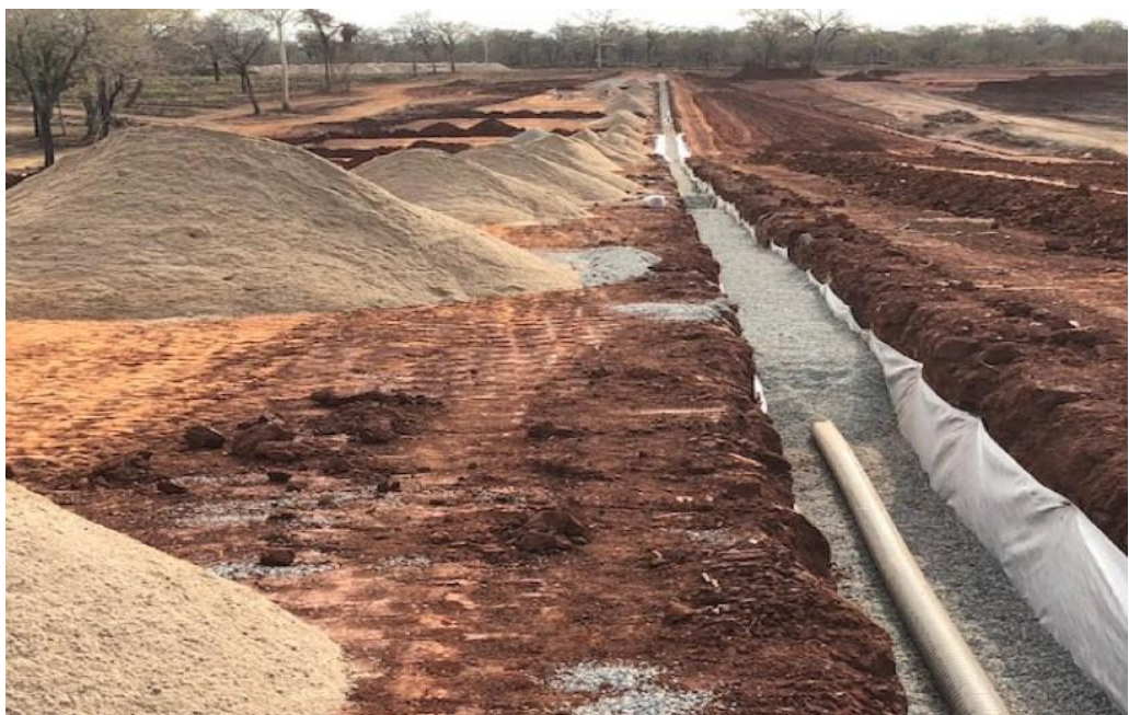
Curtain drain installation at the TSF
