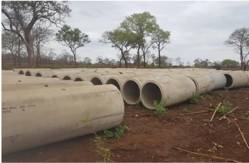
Culverts for installation to support site access through wet season
