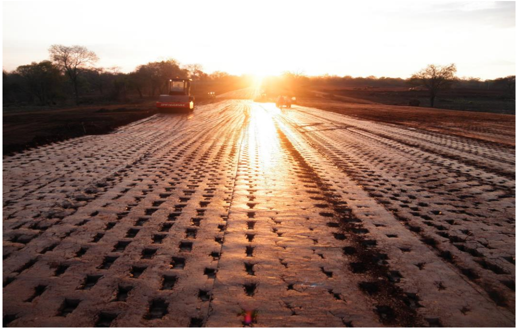
TSF wall compaction
