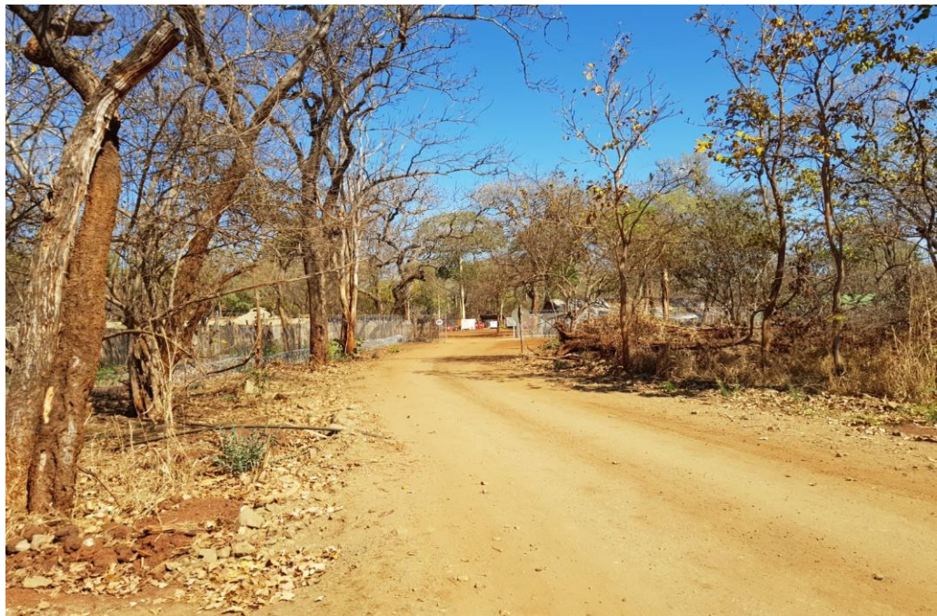
Site roads completed
