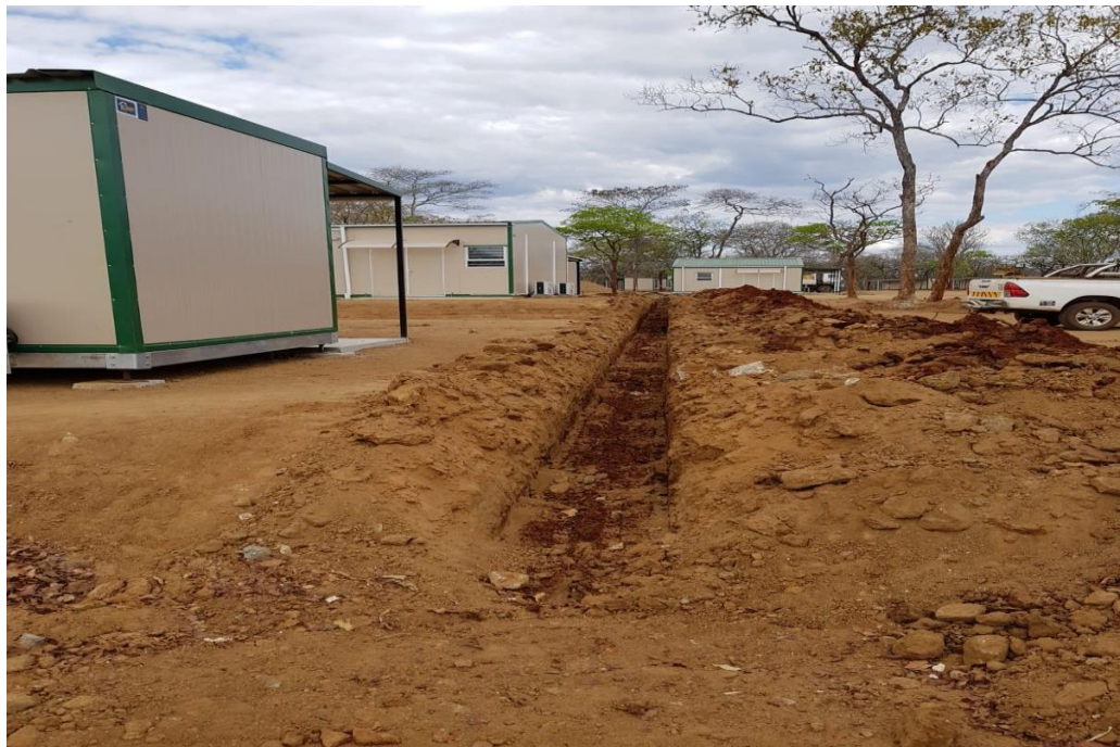
Camp sewage trenches in progress
