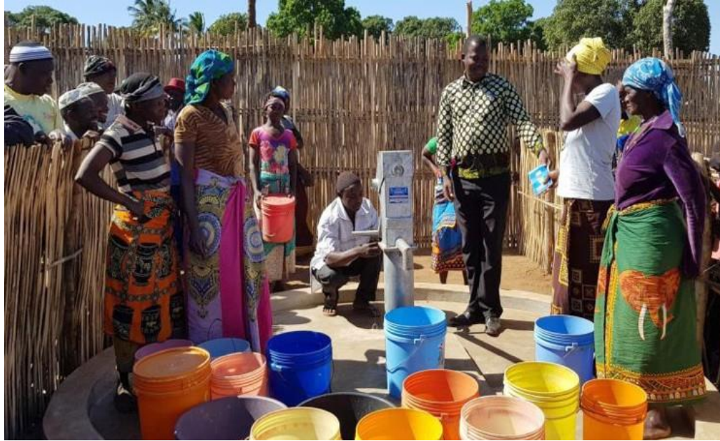
Installation of village water bore
