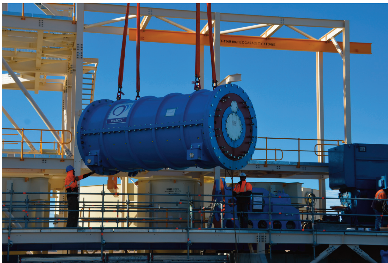
Figure 7: IsaMill™ craned into position 15 August
