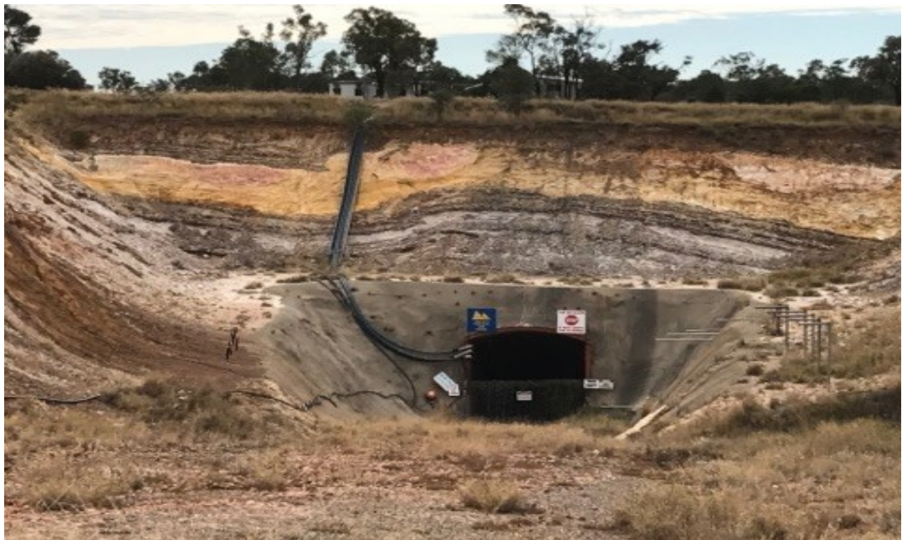
Figure 5: Portal to underground workings.
