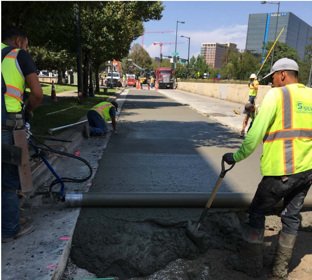
Figure 2 – One of Two New Trial Sections of Concrete Pavement in second trials
