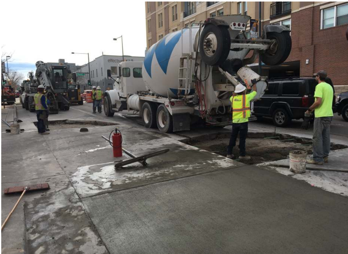
Figure 1. EdenCrete® Trial Slabs in first trials.
