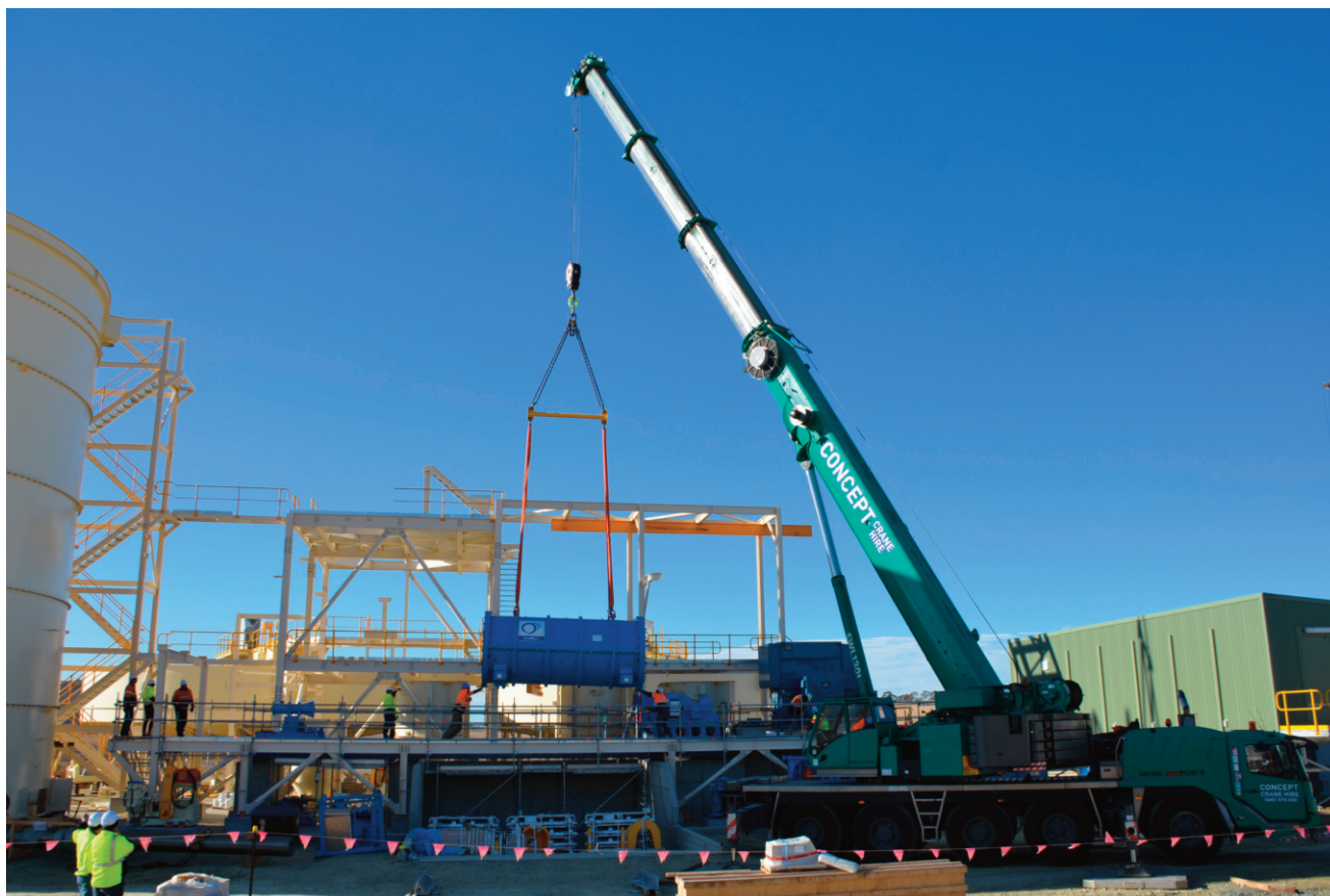
Figure 7: IsaMill™ craned into position 15 August
