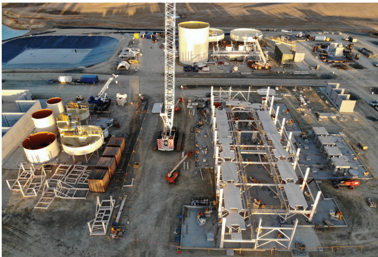
Figure 3: Concentrate storage tanks and thickener (background)
