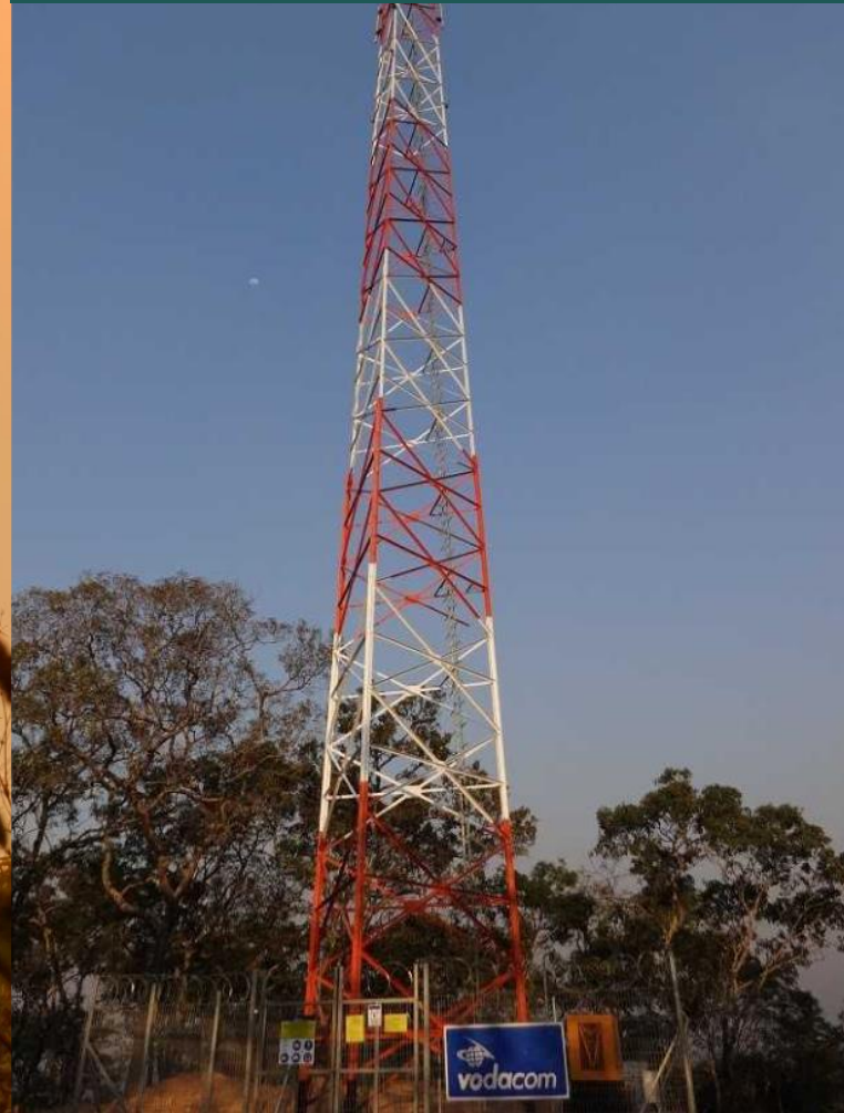
New Site Phone Tower online
