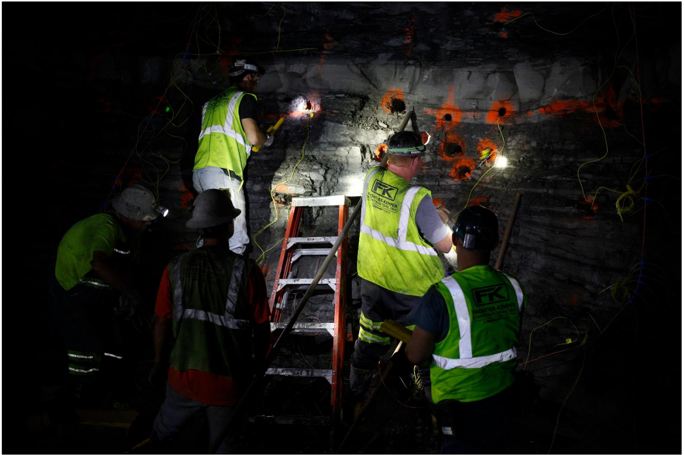
Figure 3: Preparing explosive charges to advance excavation at the decline
