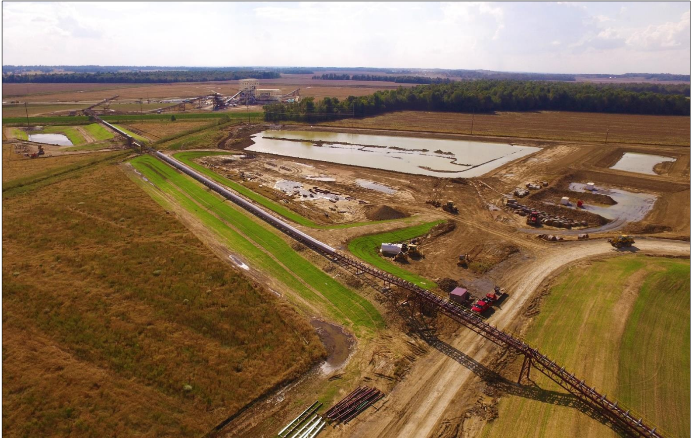
Figure 2: Overland conveyor connecting the slope portal to the CHPP
