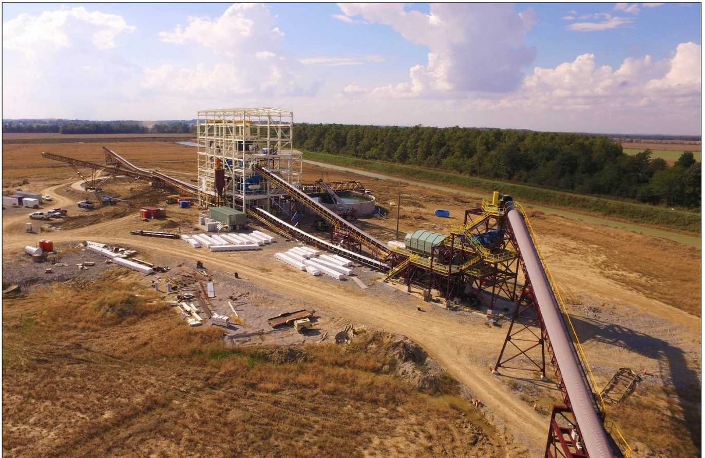
Figure 1: CHPP overview, including ROM reclaim conveyor, rock breaker structure, CHPP, thickener and stackers
