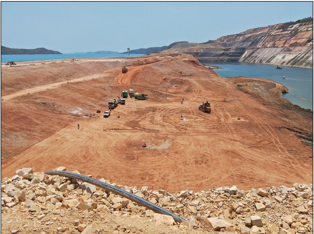
Figure 2: Re-profiling of the central inner seawall, looking west, October 2018.
