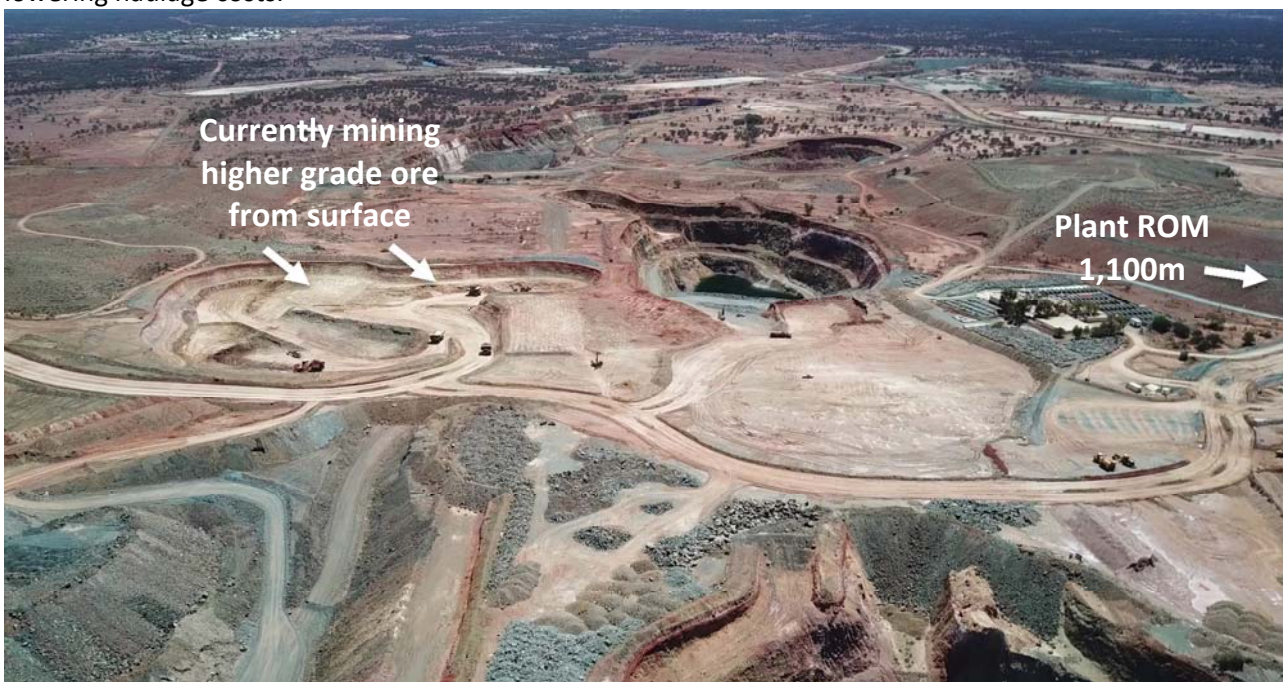
Photo 1: Mining of higher grade ore at Wiluna West Pit only 1,100m from the Wiluna gold plant
