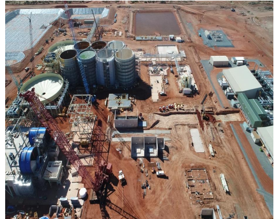
Gruyere Gold Project, Western Australia
