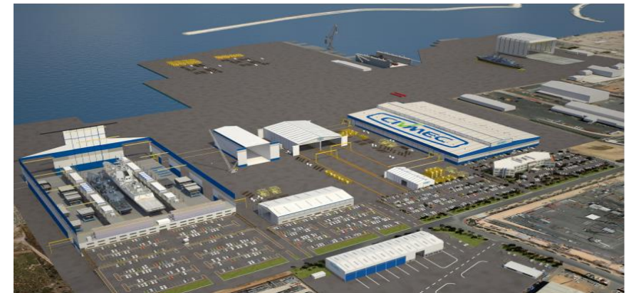
Henderson facility – showing ship assembly hall with AWD/frigate inside
