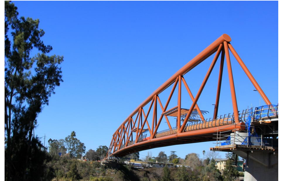
Nepean River Bridge, Penrith NSW
