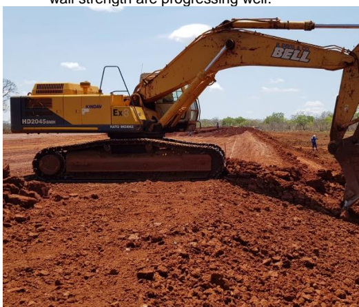
Figure 5. Montepuez Graphite Project TSF wall progressing well with excavator forming final wall angles
