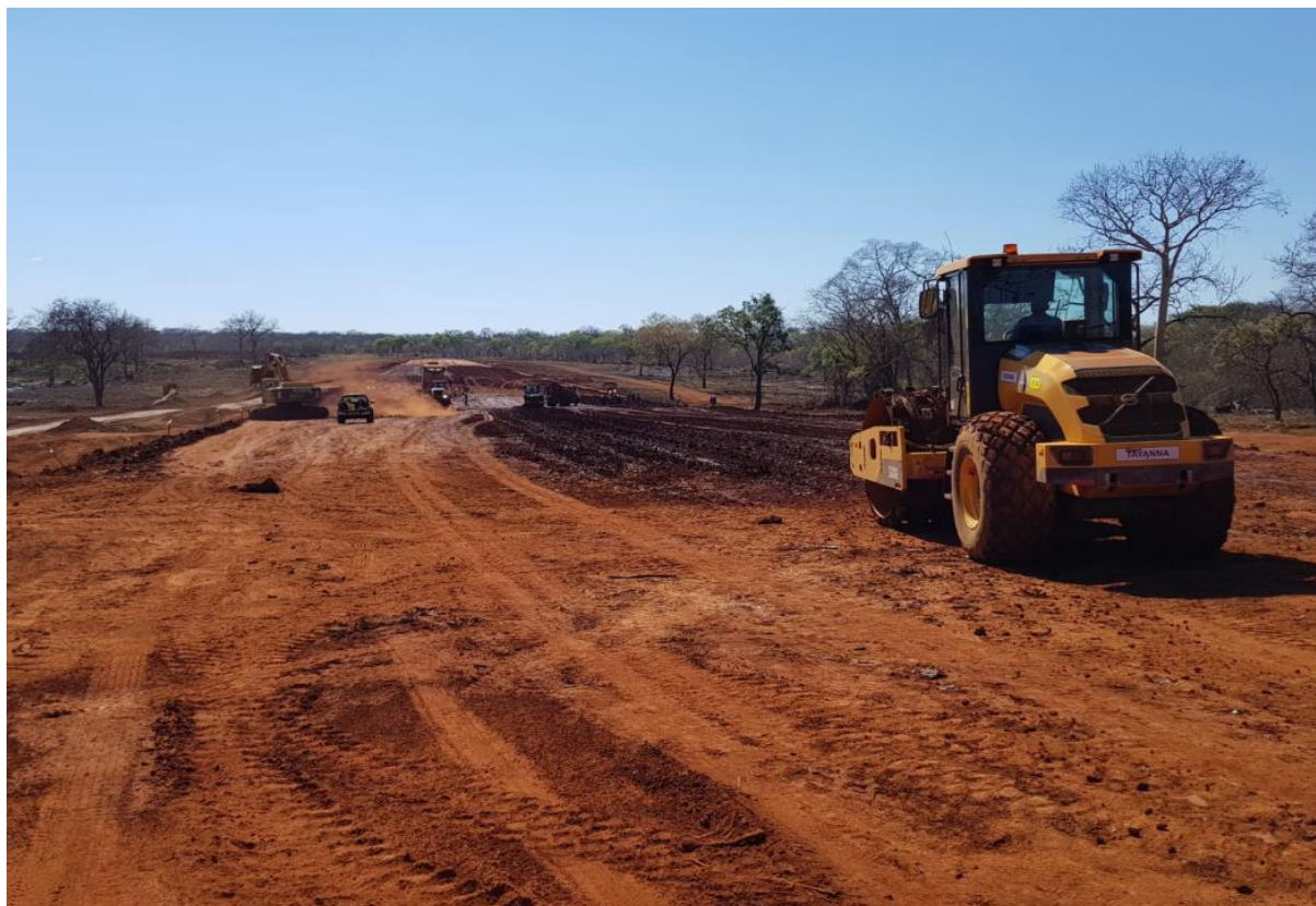
Figure 7. Montepuez Graphite Project TSF civils work, managing moisture content to ensure appropriate compaction and wall strength are progressing well.
