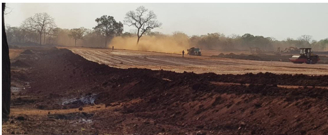
Figure 4. Montepuez Graphite Project TSF civils work, managing moisture content to ensure appropriate compaction and wall strength are progressing well.
