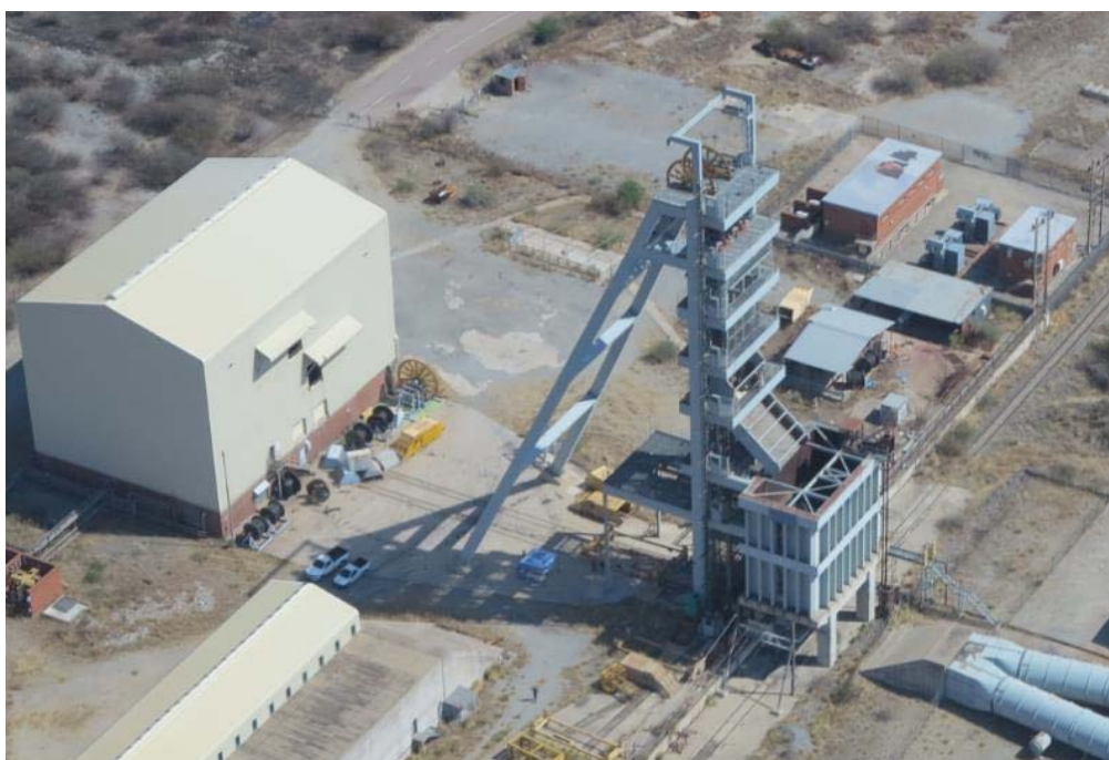
Contemporary shaft hoisting head gear and winder equipment option secured in South Africa
