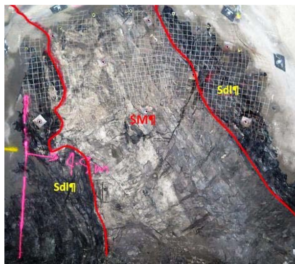
595 ore drive (4.5mW x 4.5mH) @ 9.0% Ni
