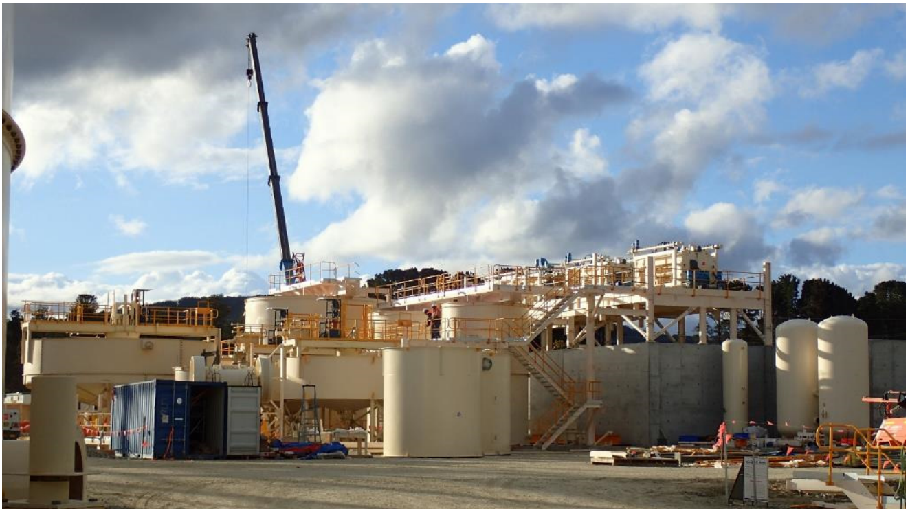
Figure 8: Concentrate handling area – filters installed above concentrate storage bunkers
