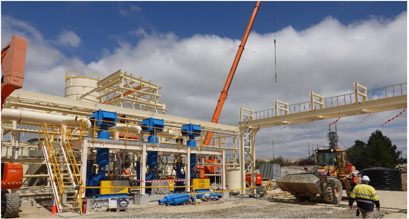
Figure 7: Flotation reagents and blower area
