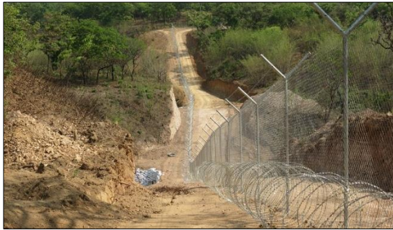
Completed fence line
