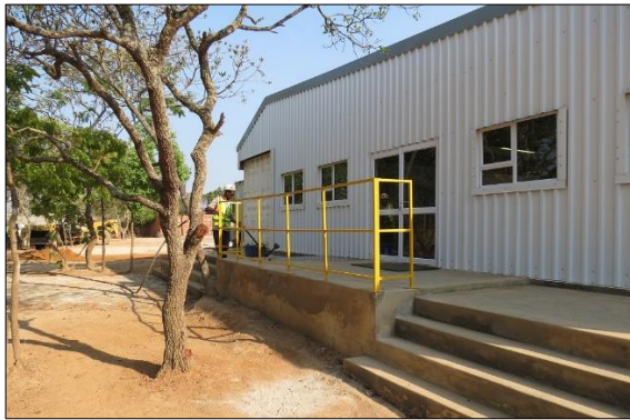
New Kitchen/ Mess Hall completed
