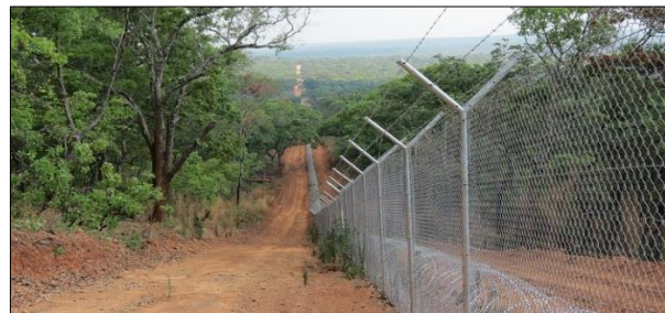
Completed fence line
