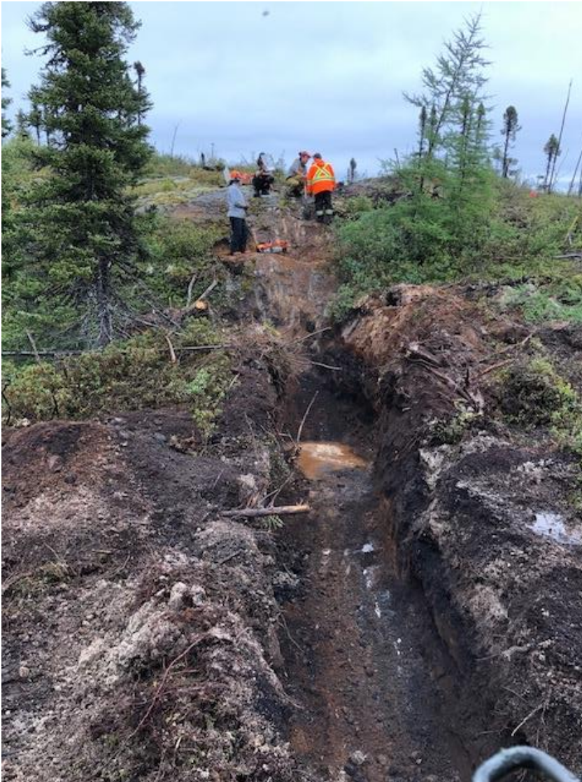
Figure 7: Trenching and sampling being undertaken at the Lac Rainy Graphite Project, Quebec
