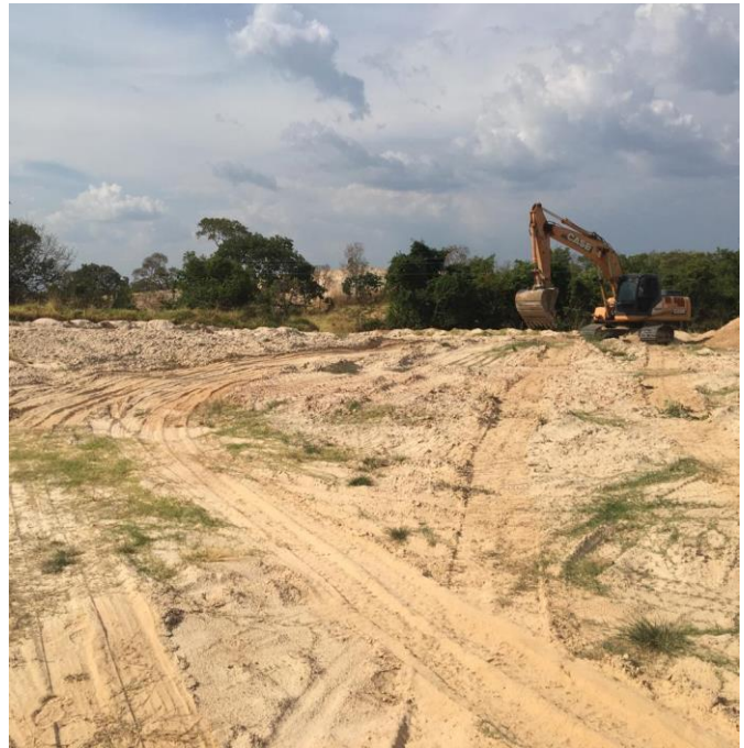
Figure 7. Tailings Stockpile 1 at Cascavel (SP 2 in background)
