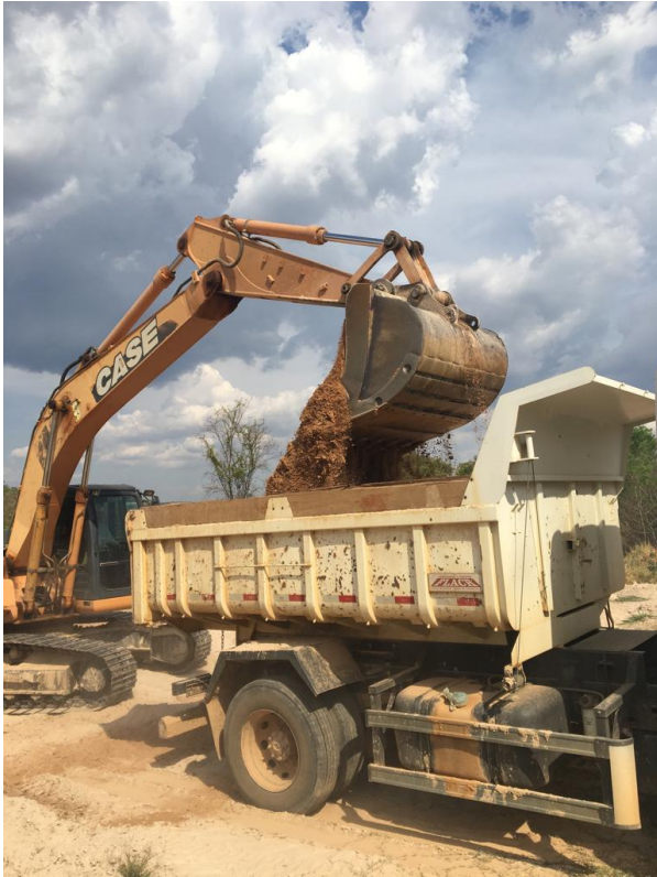
Figure 6. Tailings sample transported to third party mill
