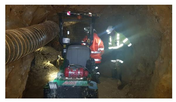
Preparation for installation of the underground power cable and auxiliary fan is underway. This
