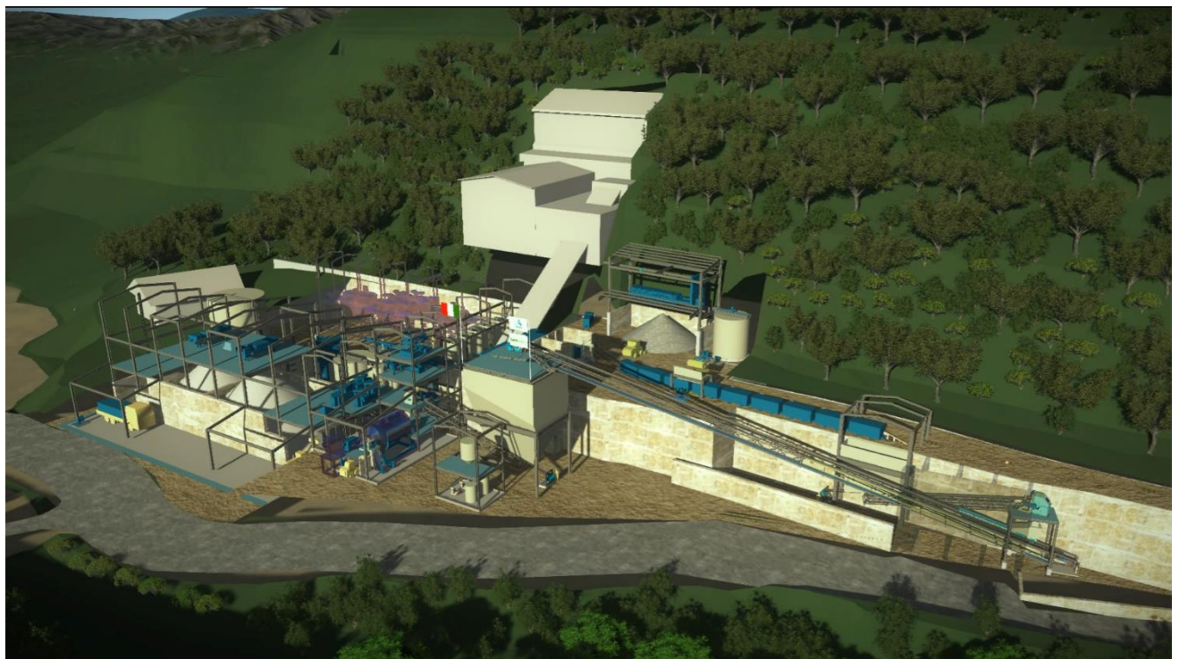
Figure 2: Processing plant layout at Riso (shed not shown) utilising rail wagons for ore & waste transport
